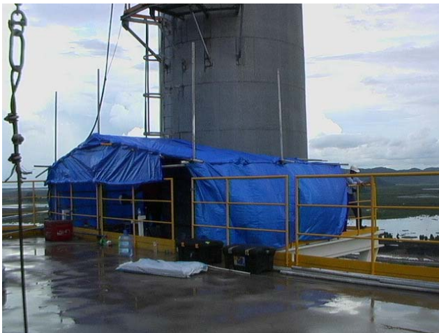
Picture 2 Stack gas sampling at the top of the preheater tower
