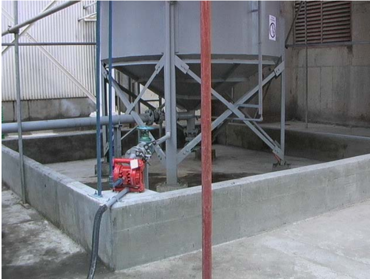
Picture 1 Storage and feeding tank for insecticide
