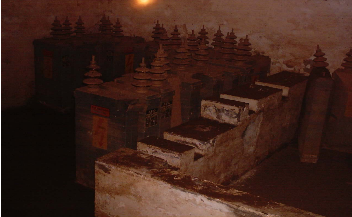
Plate 5: Decommissioned and disconnected capacitors stored at capacitor banks at Achimota
