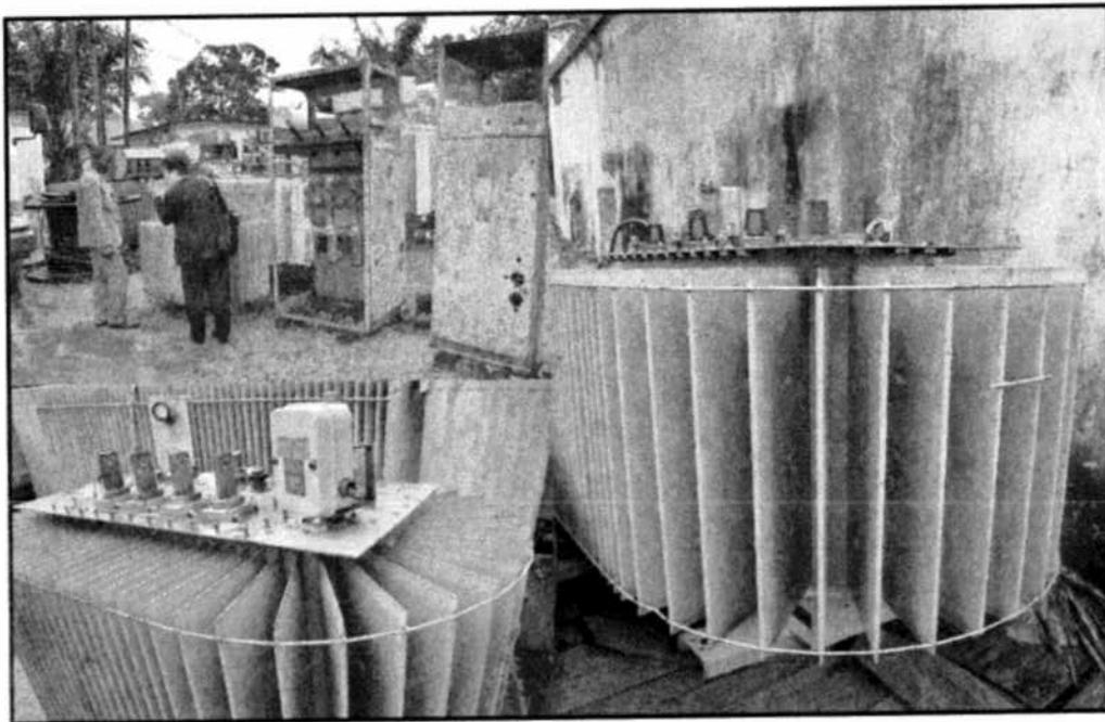
Figure 5 PCB transformers left outside without any labels on the SNE's site in Pointe Noire
