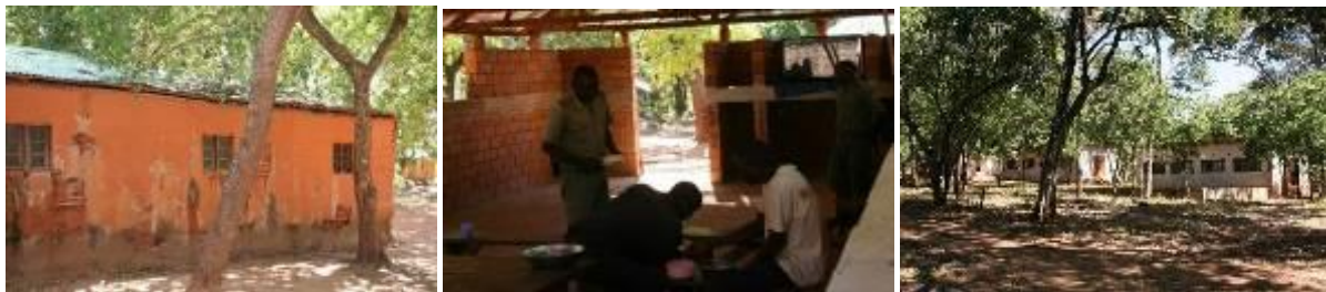
Figure A3: Staff at Mbatamila HQ of the Niassa National Reserve are separated into management and admin staff quarters, warden and scout quarters. All infrastructure is basic and progressively in decay, inadequately providing shelter from inclement weather conditions and pests. Investments supporting healthy living conditions such as mosquito proofed staff accommodation for the scout force are necessary and feasible and will contribute significantly to the NNR scouts and park management staff operational availability. In addition, investing into social infrastructure will foster team spirit and staff morale.
