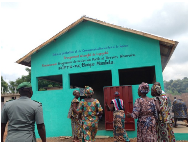
Center designed by the women's gari processing group and constructed with funds under the alternative income generation activities.
