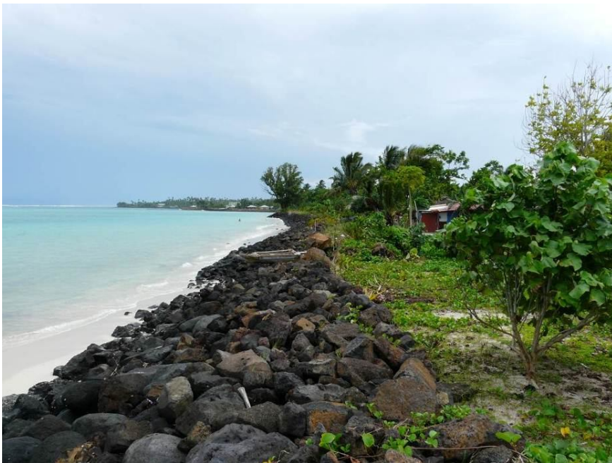
Photo 4: Part of seawall with plantings behind it.
