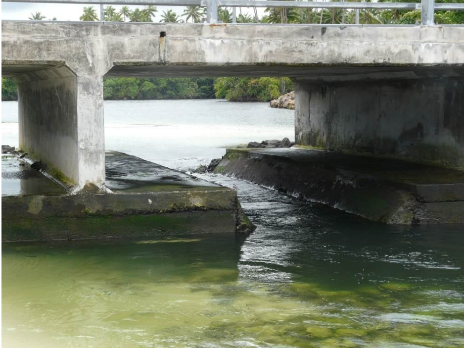
Photo 5: Bridge before mangrove wetland showing concrete removed to create channel
