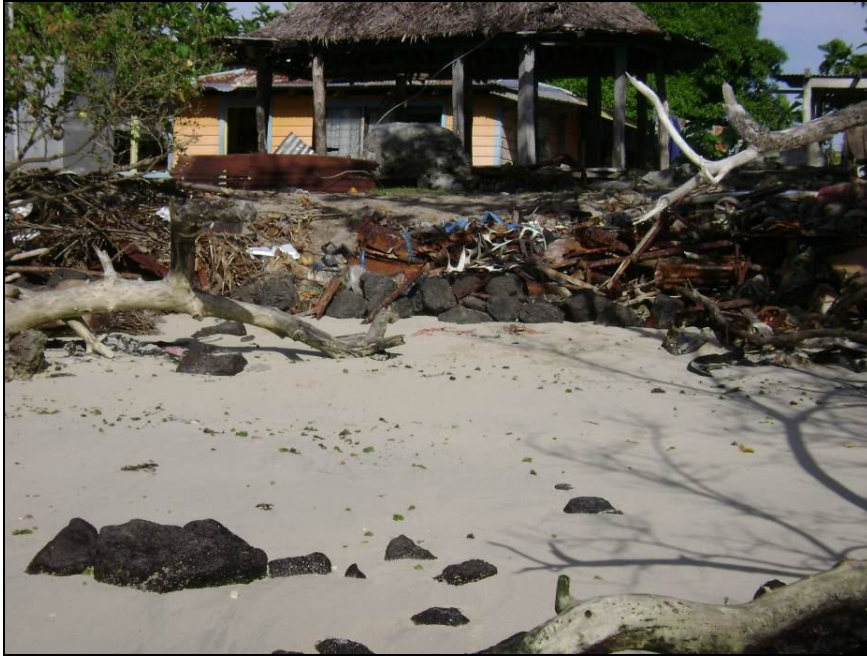
Photo: Coastal erosion at Lano pre-project (Source: LANO TAR Annex)
