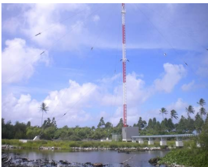
New JICA-provided AM transmitter at Funafuti
