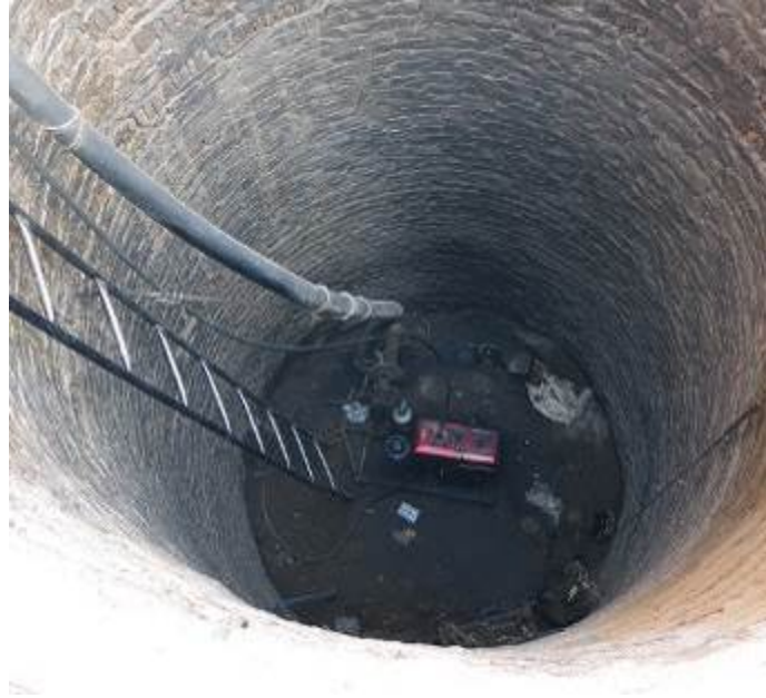
Figure 12 Typical combination dug well with driven pipe. The diesel engine and surface pump at the bottom suck water through a pipe driven into the ground (in the ground – not visible) and pump water up through the black hose shown fixed with ropes.
