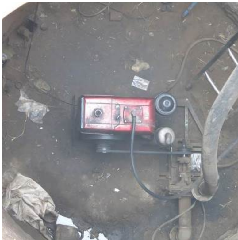
Figure 10 Typical direct drive mechanical diesel pump
