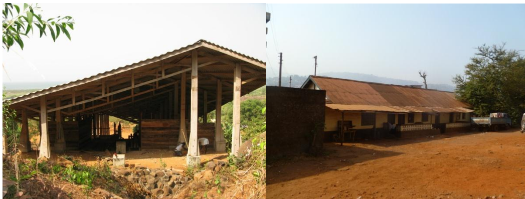
Figure 17: The Environmental and Sustainability Learning Centre of EFA at Lakka (left), and the MWR PIU house (right), both of which will benefit from RWH technologies as demonstrations underpinning trainings and political dialogues, amongst other
