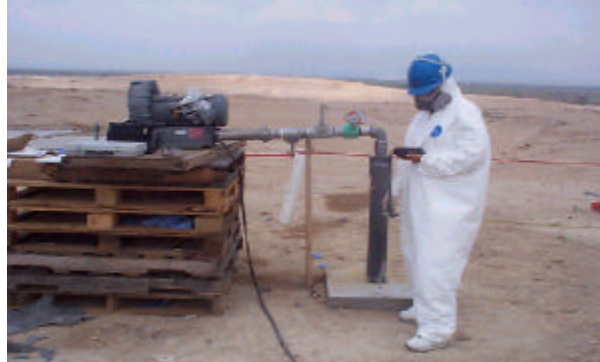
Operator Performing the Pump Test at the SIMEPRODESO Landfill
