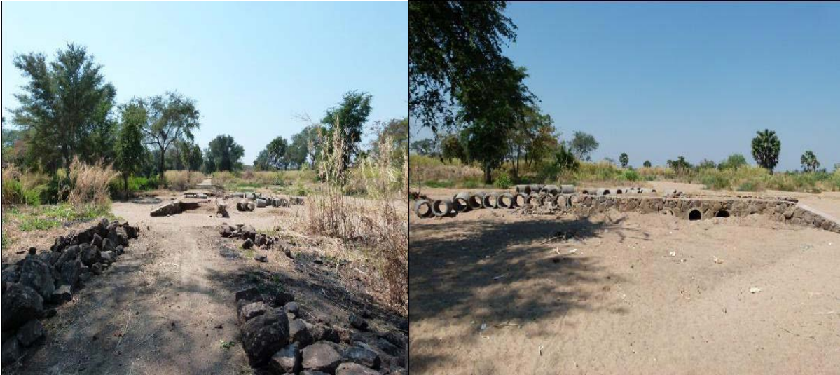
32. Figure 4: Destruction of infrastructure in Mangochi
