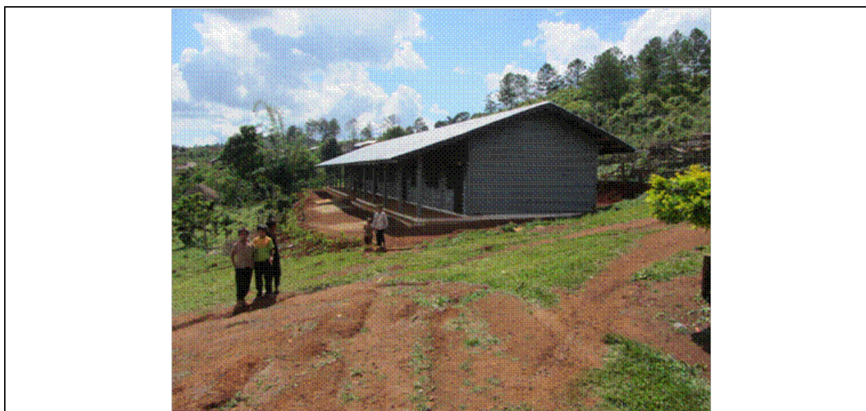
Picture 5: School infrastructure in Dakcheung district without water harvesting and storage facilities. This could be rectified providing a measure of increased community resilience to drought events.
