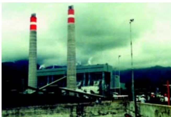
Suralaya Steam Power Plant
