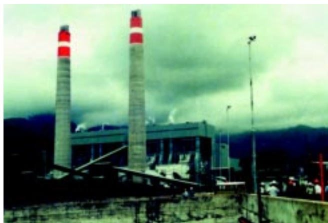
Suralaya Steam Power Plant
