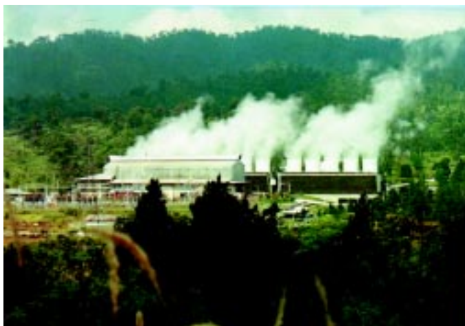
Kamojang Geothermal Power Plant
