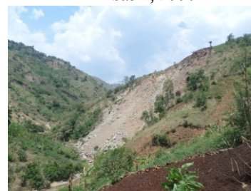
Photo 6: Land slide on the Ntakangwa river, 27 September 2013
