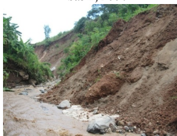
Photo 5: Land slide on the Nyabagere river, 30 March 2011
