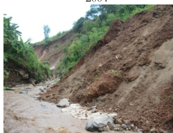
Photo 5: Land slide on the Nyabagere river, 30 March 2011
