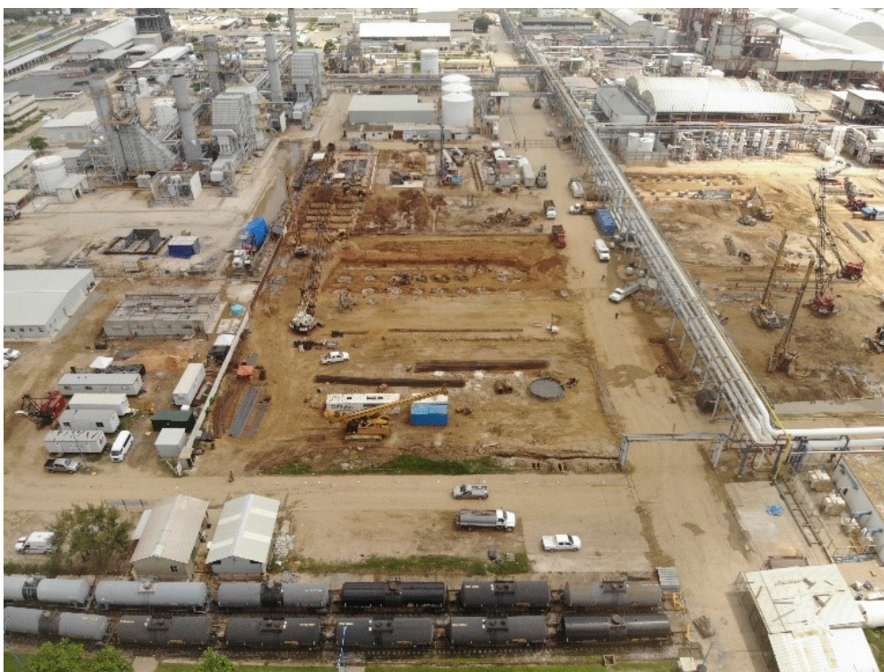
Figure 3: Overhead view of Coatzacoalcos plant construction, September 2021
