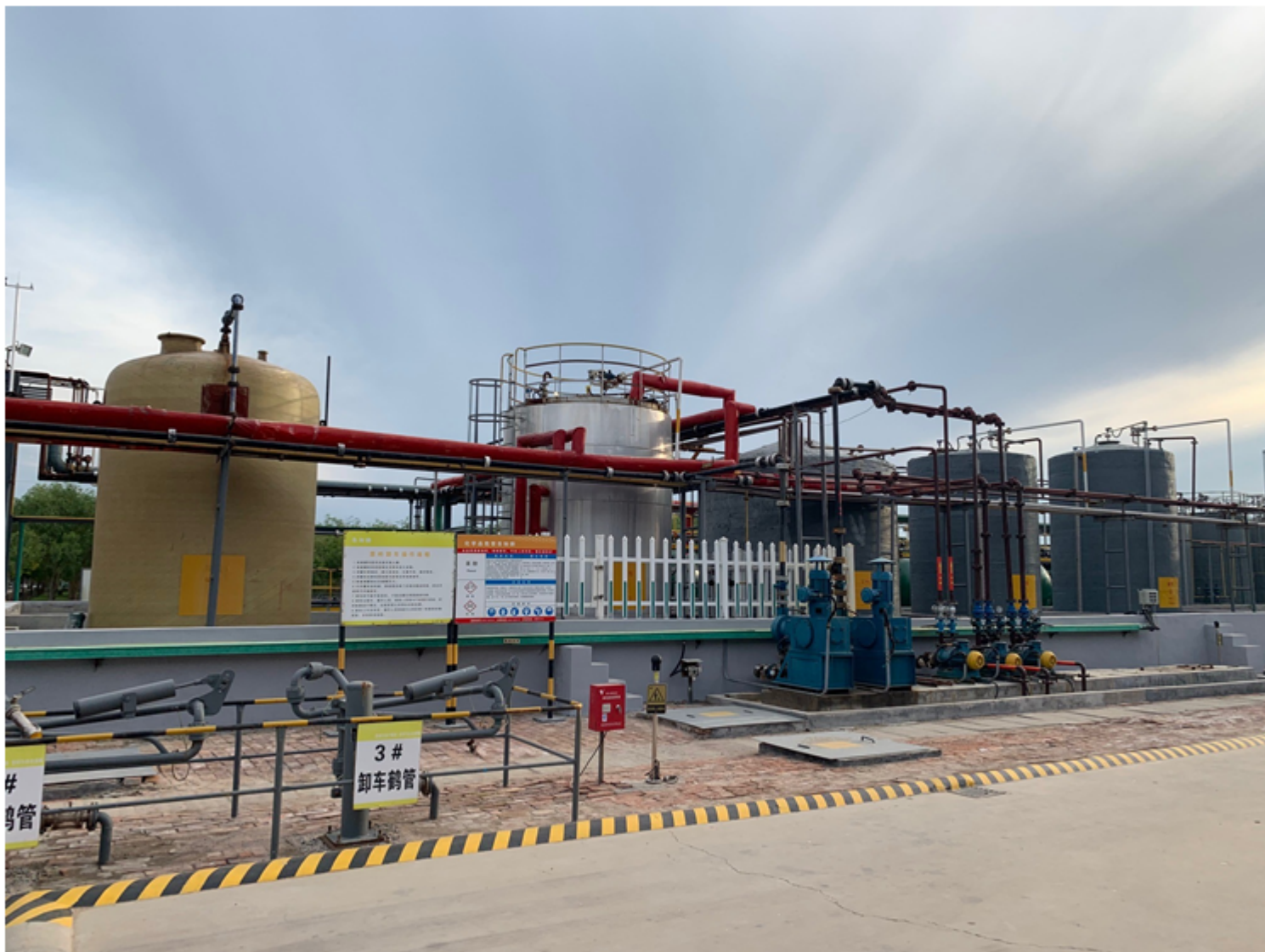
Figure 5 One of the candidate facilities for Component 2 implementation
