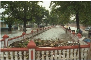
Figure 11. Agua Grande river, just before reaching the ocean in the city of São Tomé, blocked by waste and forest material dragged by the floods. Dec. 2021
