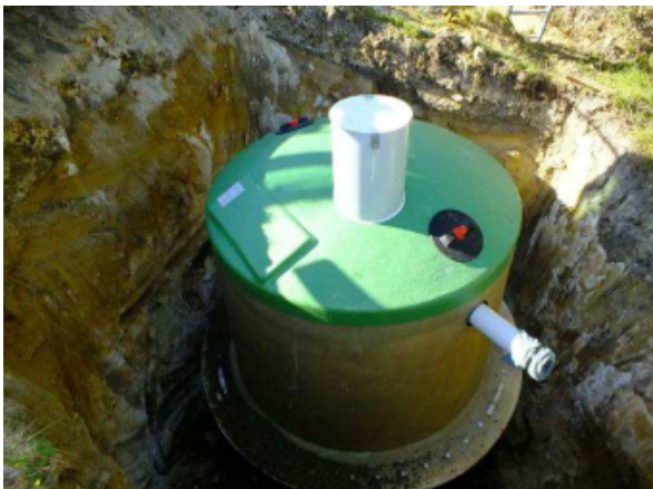
Prefabricated fibreglass system in New Zealand
