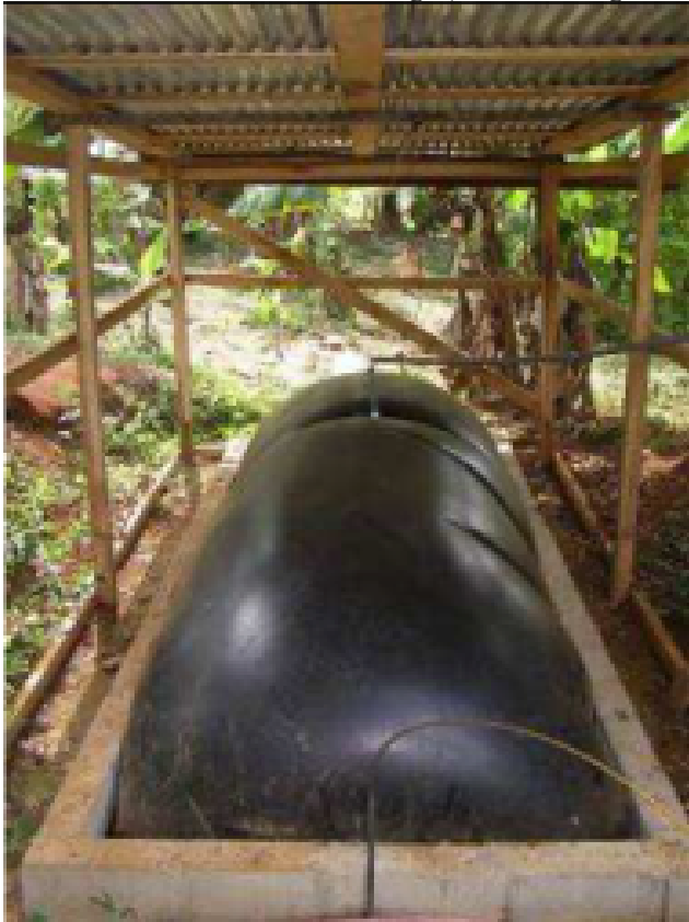
Polyethylene bag digester in Costa Rica
