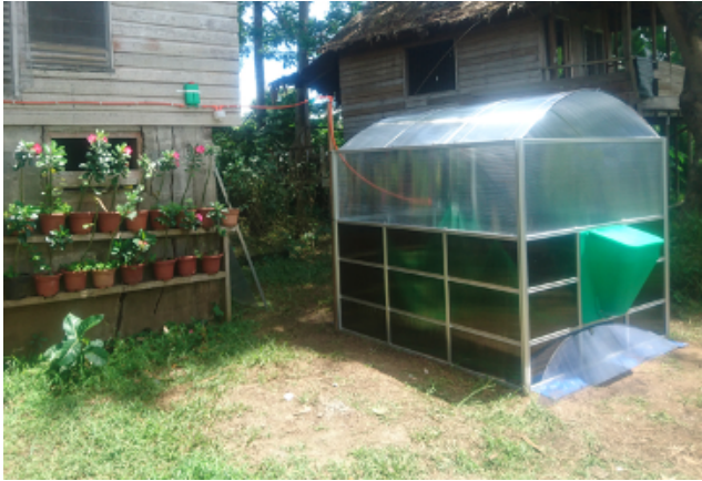
Prefabricated HDPE SupSup Biodigester in Solomon Island
