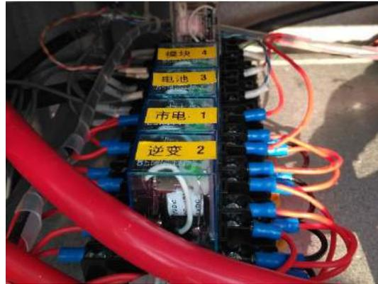
Relay 1 and 2 each control a three-phase AC contactor, while relays 3 and 4 each control two DC contactors (for positive and negative rails). Relay 2 and Relay 3 are driven by PLC control signal 1 which is enabled during standalone mode; while Relay 1 and 4 are driven by PLC control signal 2, which is enabled during grid-connected mode.
