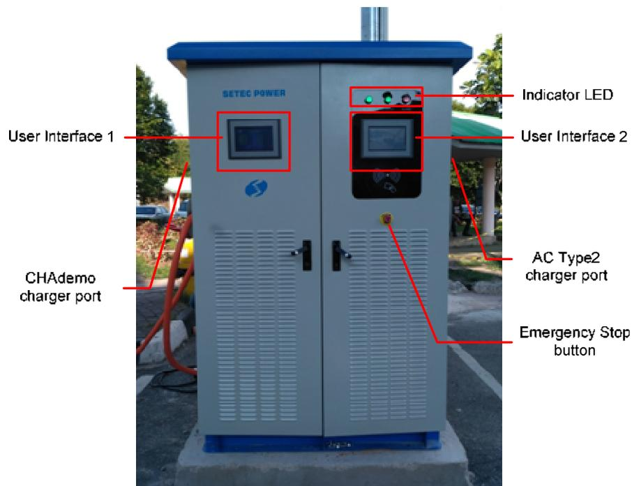
Figure above shows the front view of the EV charger system. The components and their functions are given in the table below:
