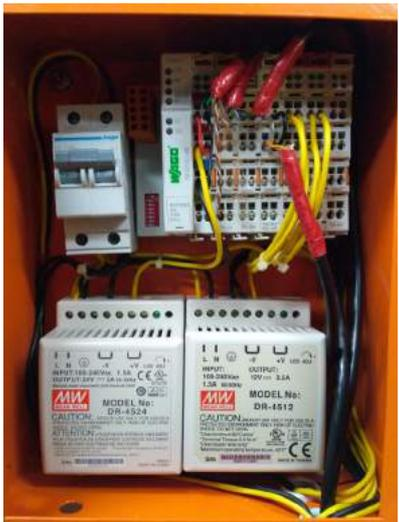
Figure 6 Wago controller module with power supplies.
