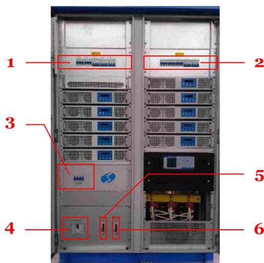
Several circuit breakers (MCCB) are used to connect/disconnect the external components to the charger system, and to provide/disconnect power supply to the subcomponents in the system. The functions of the circuit breakers are as follows:
