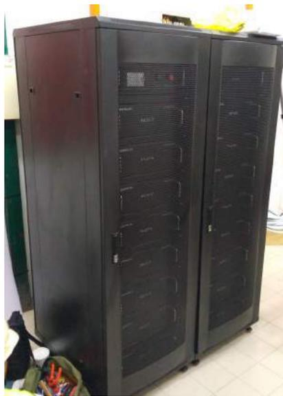
Figure 4 Lithium Iron Phosphate (LiFeSO<sub>4</sub>) 50kWh battery pack.
