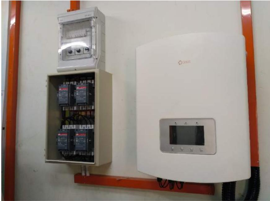
*Figure 2: Solis grid-connected inverter (right), DC contactors box (bottom left) and PV combiner box (top left) installed in the main switch board room at R&R Ayer Keroh.*
