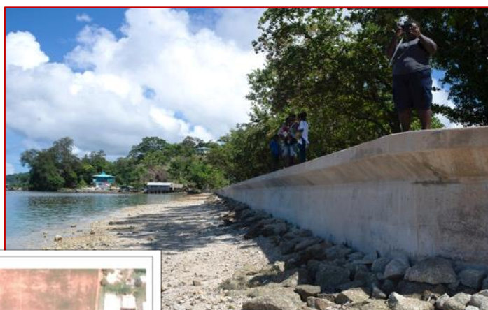
Left: Situation after investment. Road protected by a rock armor revetment, including a concrete ramp and a repaired drainage culvert.
