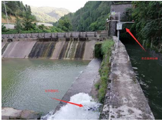
Ecological flow discharge and online monitoring equipment in Chongqing Taiping SHP Station
