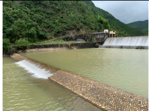
Ecological dam beneath Fujian Gaofang Stage II SHP Station
