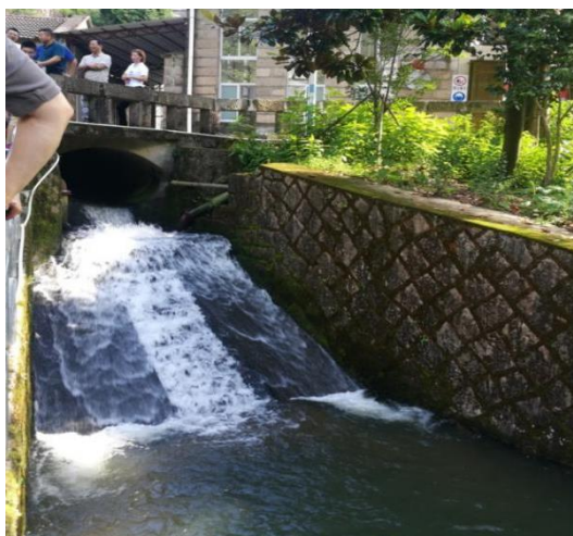
Fig. 3.22 Minimum Flow Discharge and Its Monitoring, Restoration of River Bank Land of Panxi Cascade Hydropower Plant
