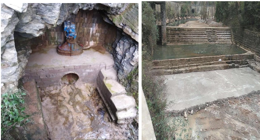
Fig. 3.35 Minimum Discharge Valve and Ecological Weir of Jingtanfeng/Huangyan Hydropower Plant
