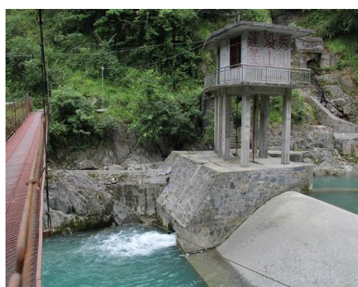
Fig. 3.42 Minimum Discharge of Xinpingya Hydropower Plant
