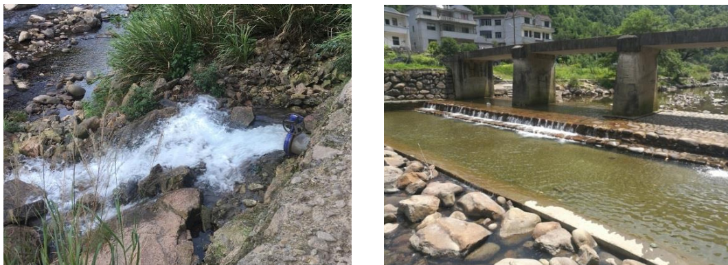
Fig. 3.21 Minimum Discharge and Ecological Weir of Qingshuitan Hydropower Plant
