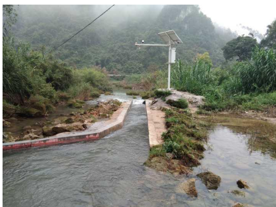
Fig. 3.30 Minimum Discharge and Its Monitoring of Sandieling/Dongpai Hydropower Plant
