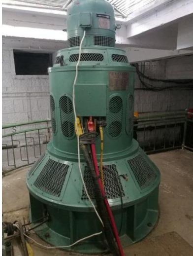
Fig. 3.38 Ecological Unit and Minimum Discharge of Mabozi Hydropower Plant
