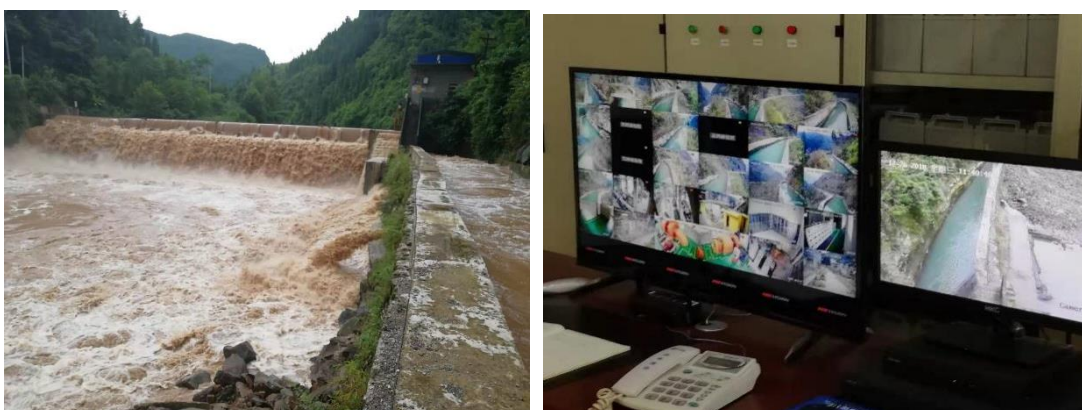
Fig. 3.36 Minimum Discharge and Its Monitoring of Taiping Hydropower Plant
