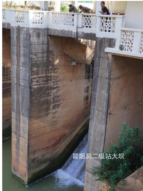
Fig. 3.37 Minimum Discharge of Maoyandong Cascade II Hydropower Plant
