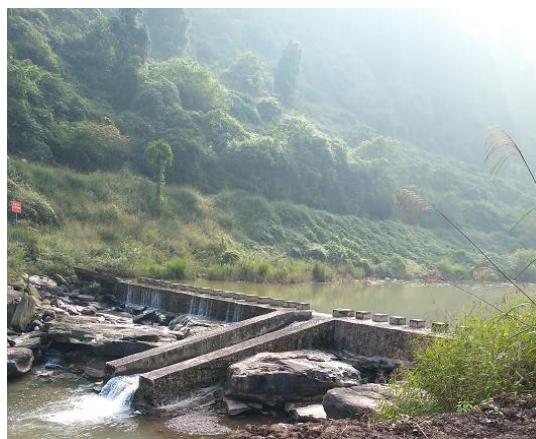
Fig. 3.32 Minimum Discharge and Ecological Weir of Majing Hydropower Plant
