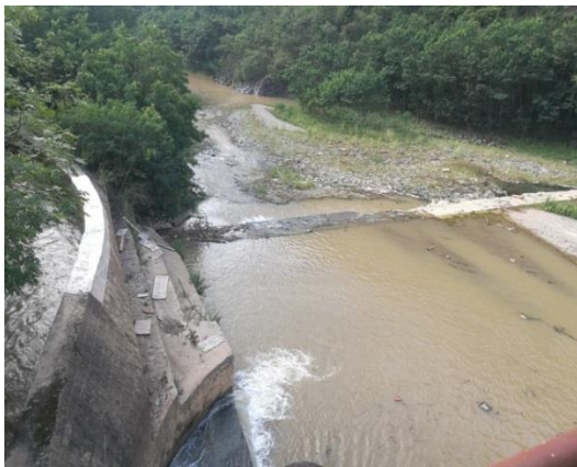
Fig. 3.39 Minimum Discharge and Ecological Weir of Chahe Hydropower Plant
