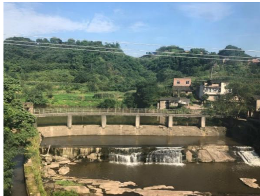
Fig. 3.33 Ecological Weir of Xiaokeng Hydropower Plant
