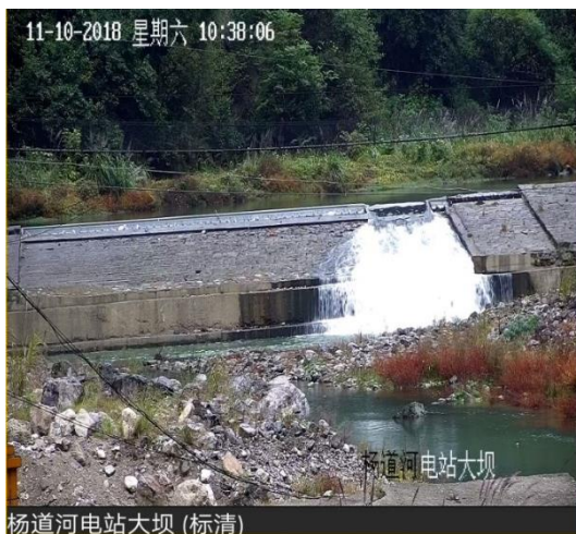
Fig. 3.27 Minimum Discharge and Its Monitoring of Yangdaohe Cascade Hydropower Plant (Yangdaohe)
