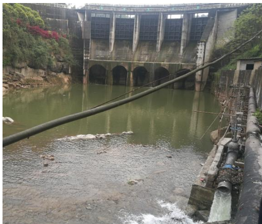
Fig. 3.32 Minimum Discharge and Ecological Weir of Majing Hydropower Plant
