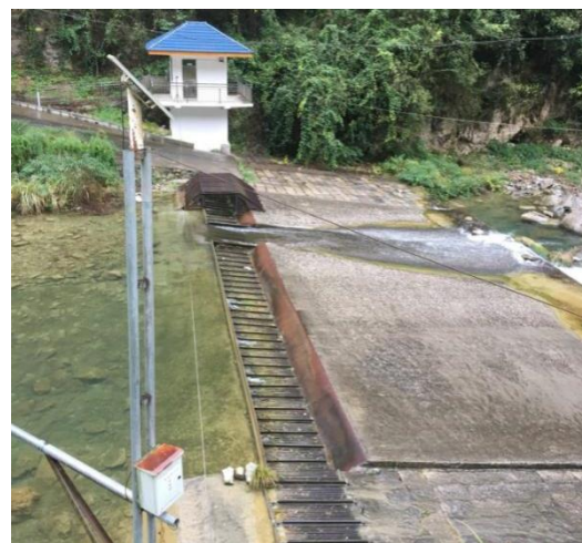
Fig. 3.27 Minimum Discharge and Its Monitoring of Yangdaohe Cascade Hydropower Plant (Yangdaohe)
