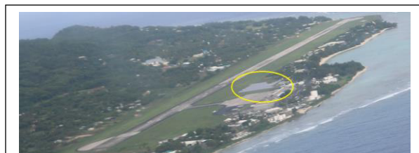
Figure 1. Photo taken in 2016 showing existing PV installation (inside yellow ring).
