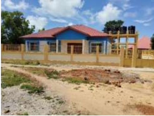
Picture 1: Internet center and water tower
