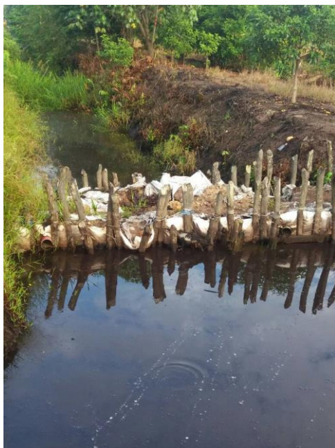
c) Canal blocking construction
