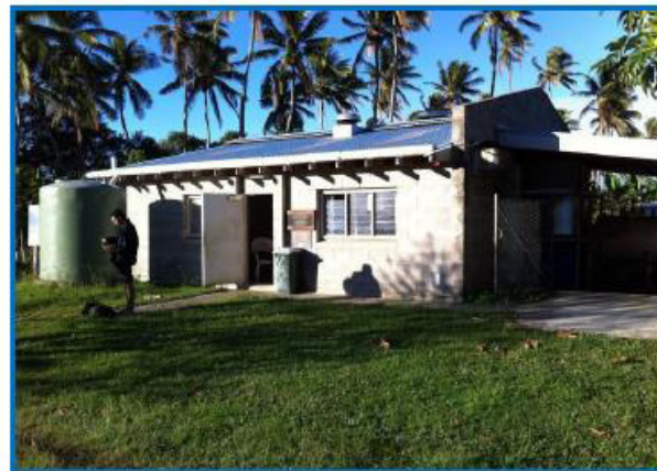
Image 2b: View of Proposed site beside existing Generation Plant
