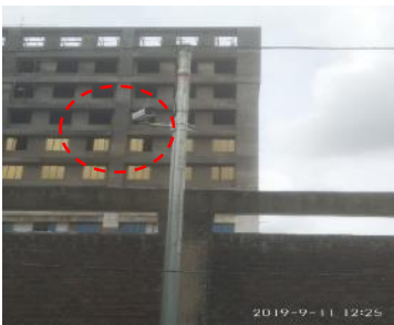
ITS - CCTV cameras installed at parking locations (MBMC)
