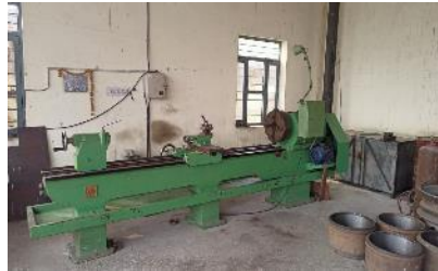
Lathe machines amongst other equipment installed
