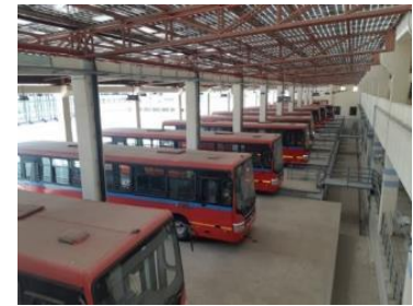
At grade depot (100 buses) with Solar PV roof, inter-connected pits next to inventory storage at Ghodbunder Depot, MBMC
