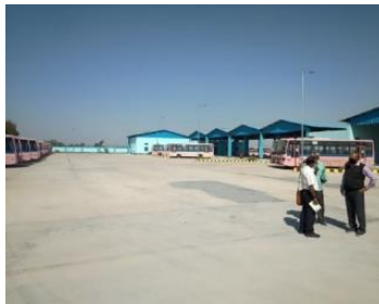
Two-level bus depot (130 bus capacity) with ETP, rainwater harvesting at Bagrana, Jaipur
