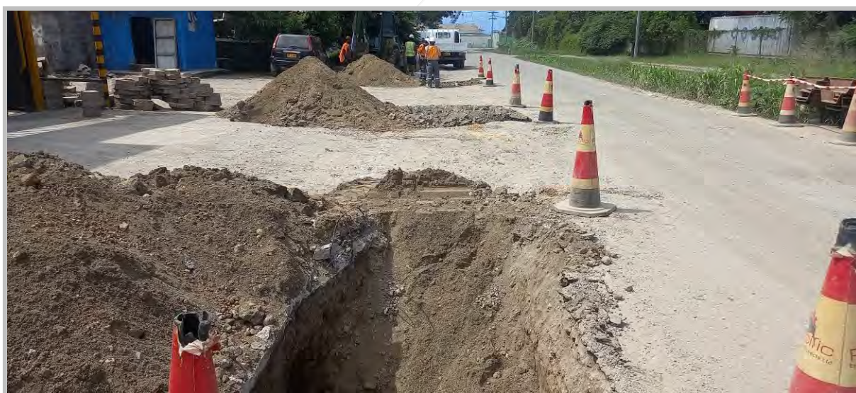
Figure 1 Ranadi-Goodwood - Potholing to expose PVC pipe encroachment on sewer alignment (Photo 13/12/23)
