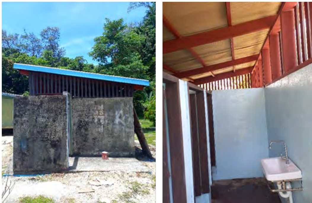
Photo 19 - Rehabilitated Roof and New Handbasins McMahon Primary School
