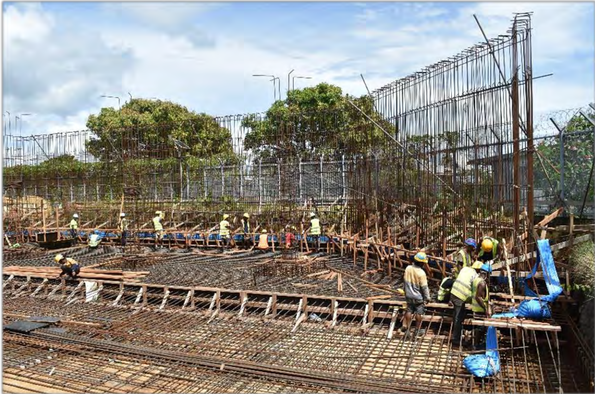
Figure 5 Steel fixing at Tasahe Tank (Photo 1/11/23)
