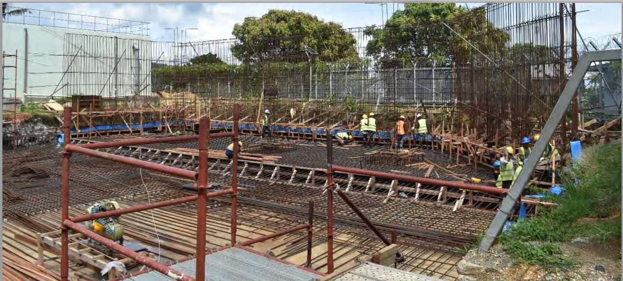
Figure 5: Steel Fixing and Formwork at Tasahe Reservoir Site (Photo 1/11/23)
