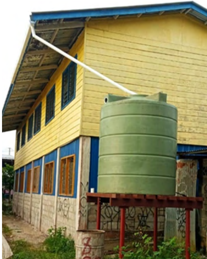
Photo 26 - Sinasu rainwater collection system
