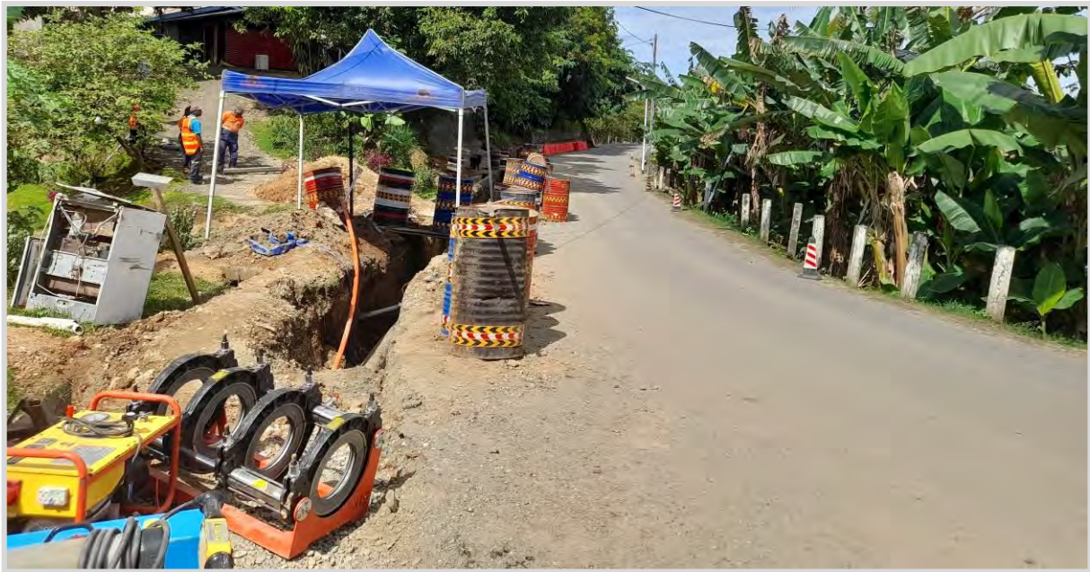
Figure 4 Trunk Mains – Trenching at East Kola (Photo 6/11/23)
