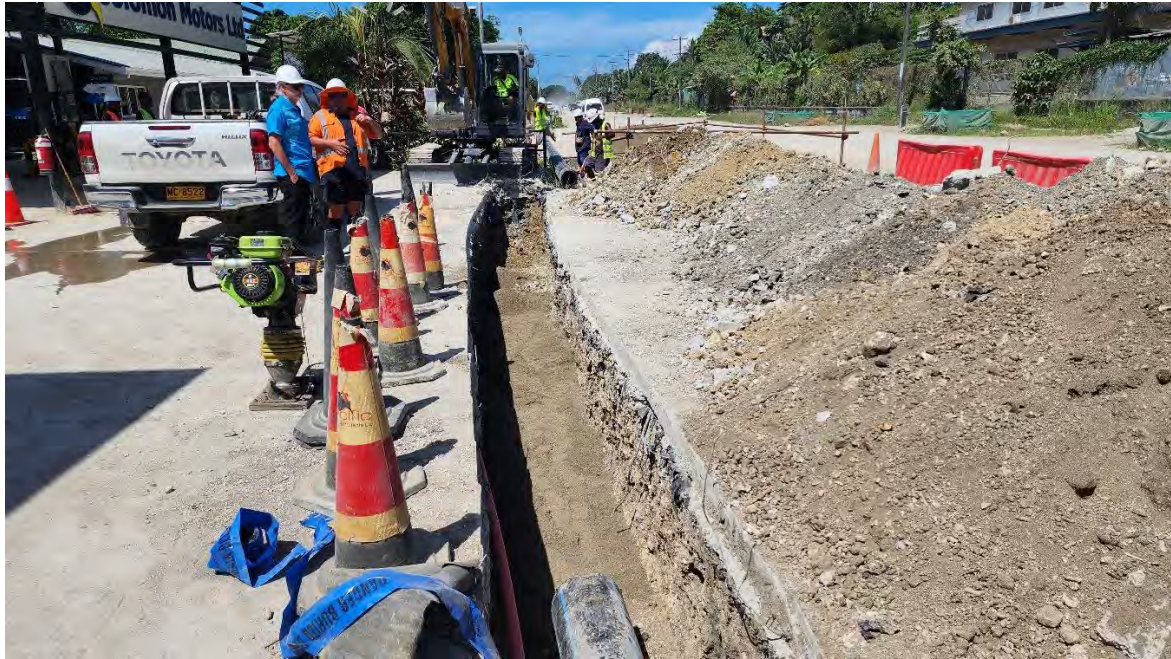
Figure 3 Pipe trenching at Solomon Motors fuel station, White River (Photo 24/04/24)
