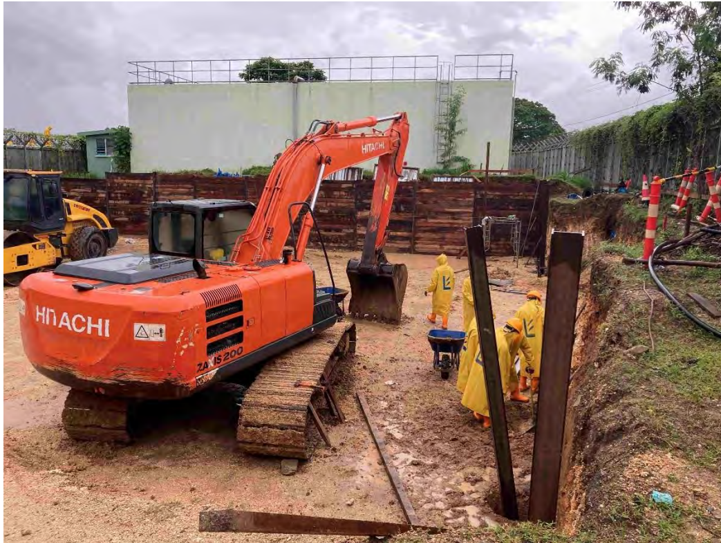
Figure 5 Shoring Work at Panatina Tank Site (Photo 29/01/24)
