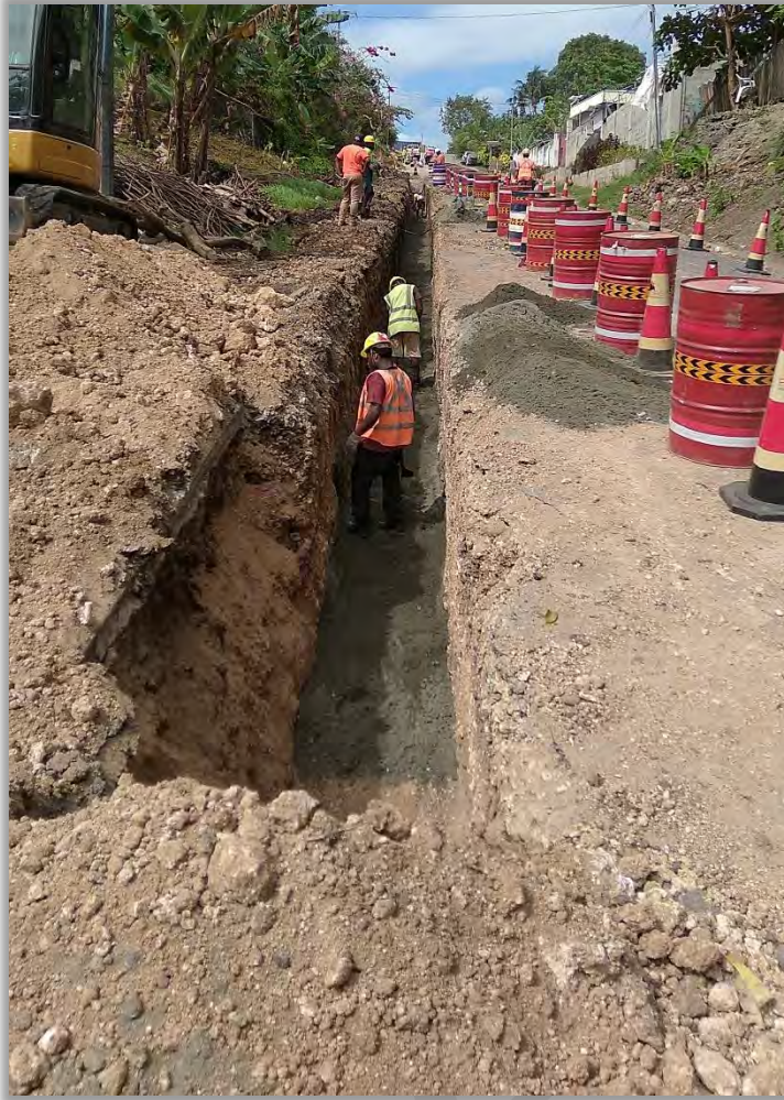
Figure 3: Trenching at Lower Tanakake Road, Panatina (Photo 7/09/23)
