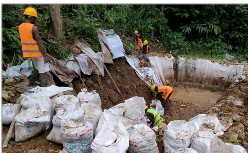
Figure 2 Sediment Pond Works at Kongulai WTP Site (Photo 16/11/23)
