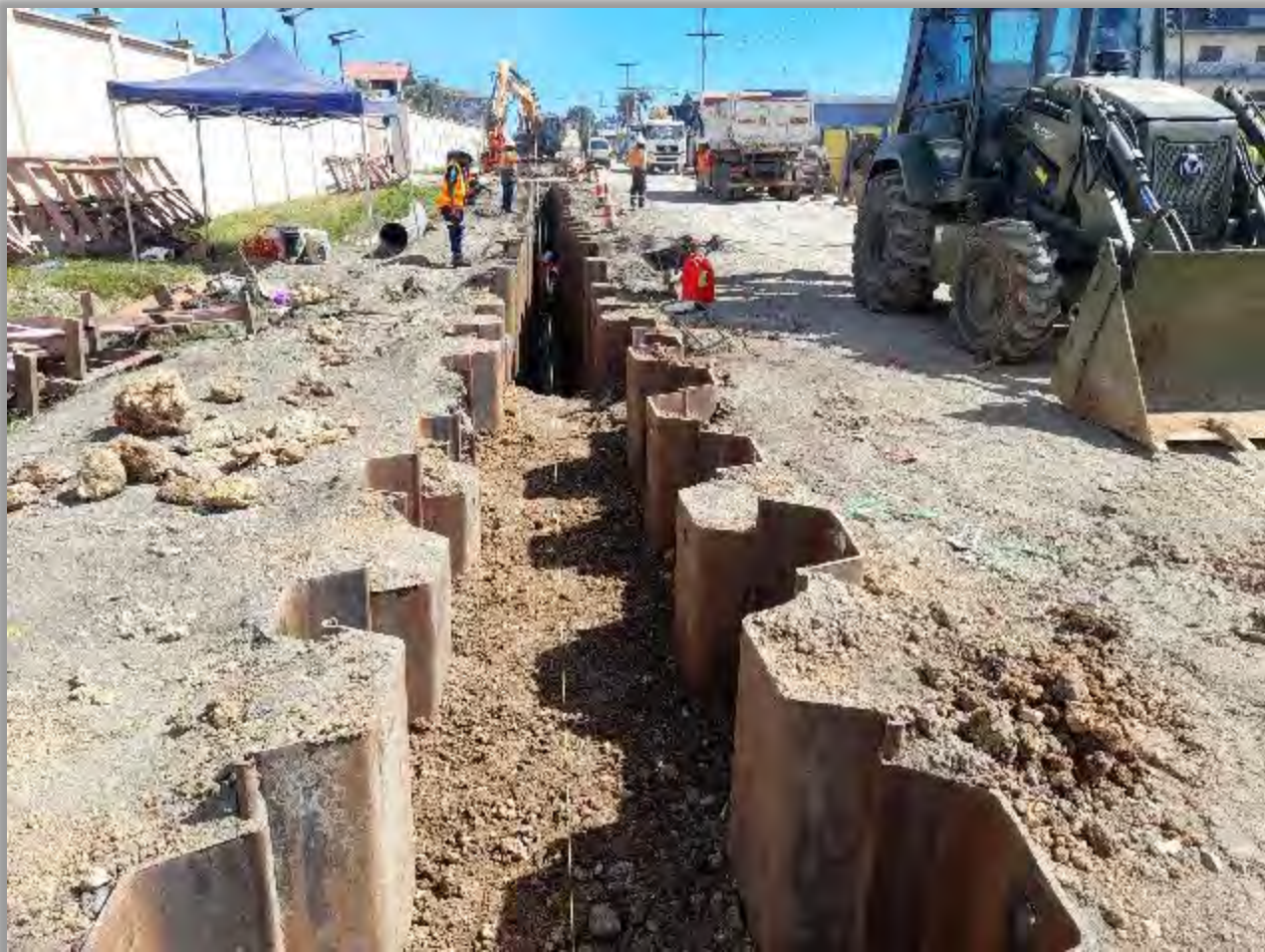
Figure 7: First section of pipe laid, 24m near Ela Motors (Photo 16/08/23)
