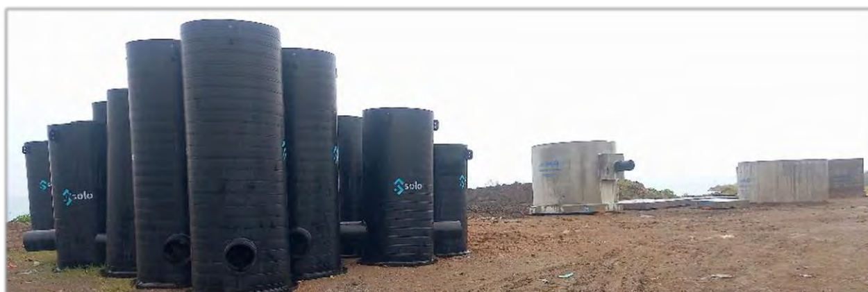
Figure 7 Goodwood Sewer PE manholes and pre-cast concrete chambers for pump station (Photo Dec 2024)
