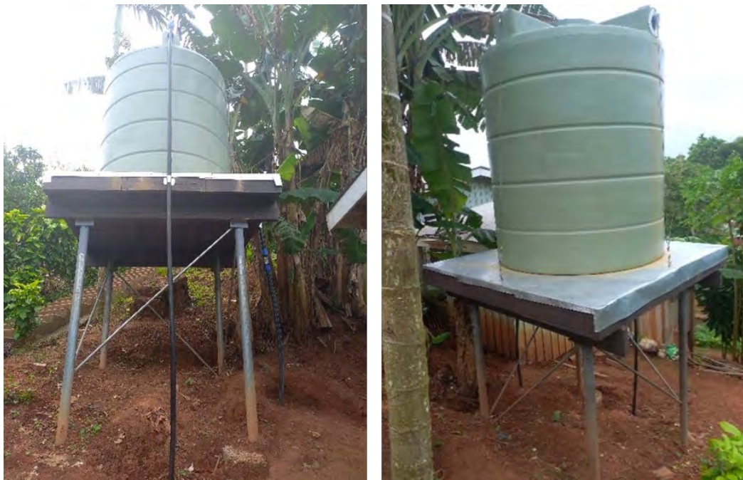
Photo 9 - Two new elevated water tanks
