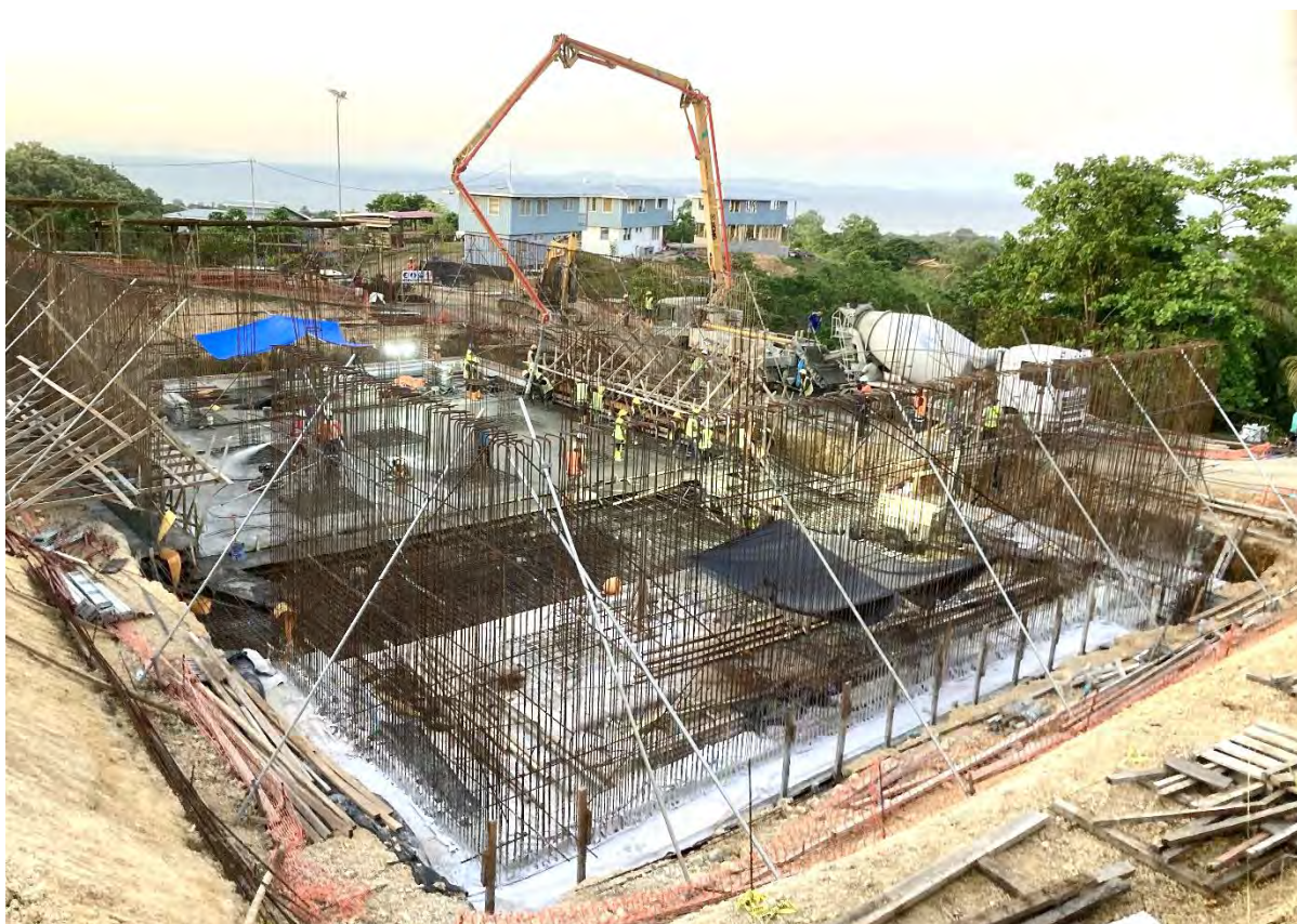
Figure 4 Titinge Tank Floor Slab Concrete Pour (Photo 24/03/24)
