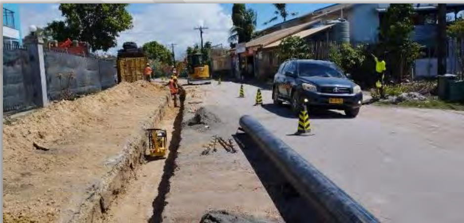
Figure 4: Compacting backfill, Panatina (Photo 2/08/23)
