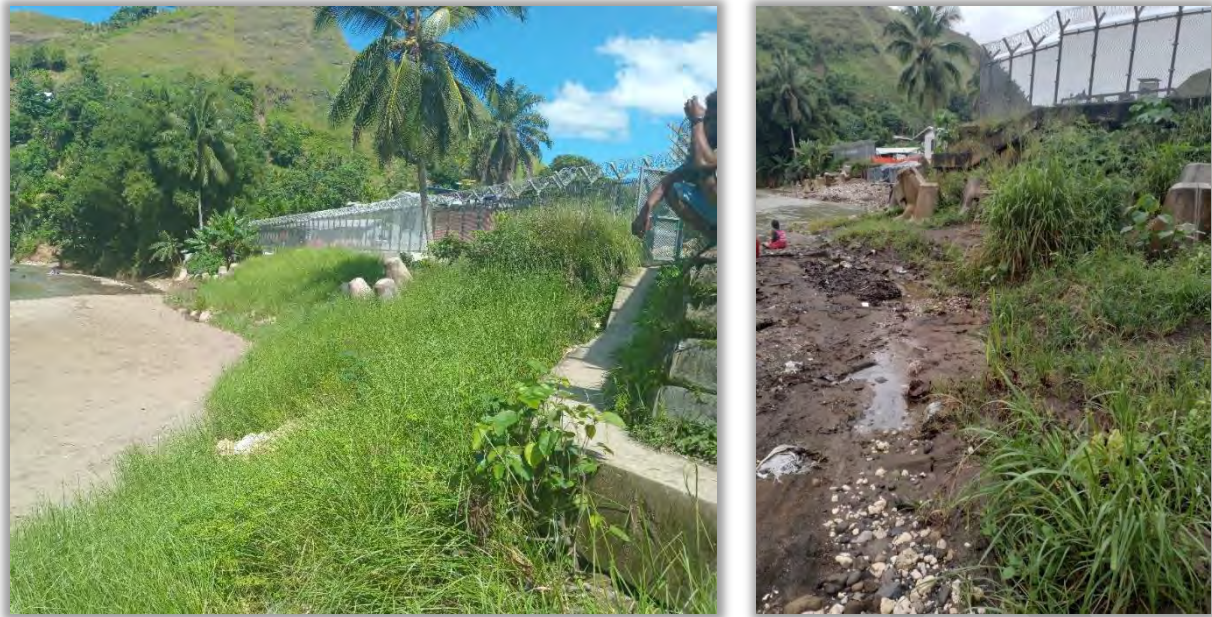
Figure 8 Tuvaruhu Erosion Protection After and Before Vetiver Grass Planting (Photos 28/02/23 Left & 29/11/23 Right)
