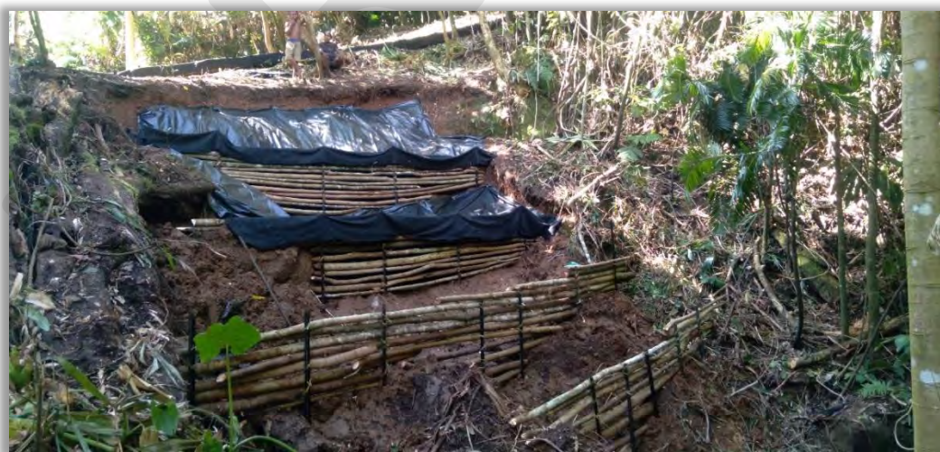
Figure 10: Temporary retaining of barrier stages with local materials (Photo 7/06/23)
