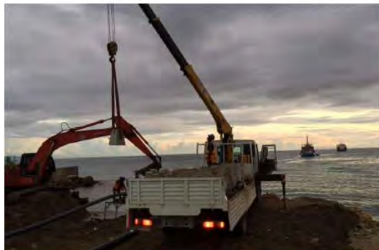
Laying of pipes at the Rove Outfall.
