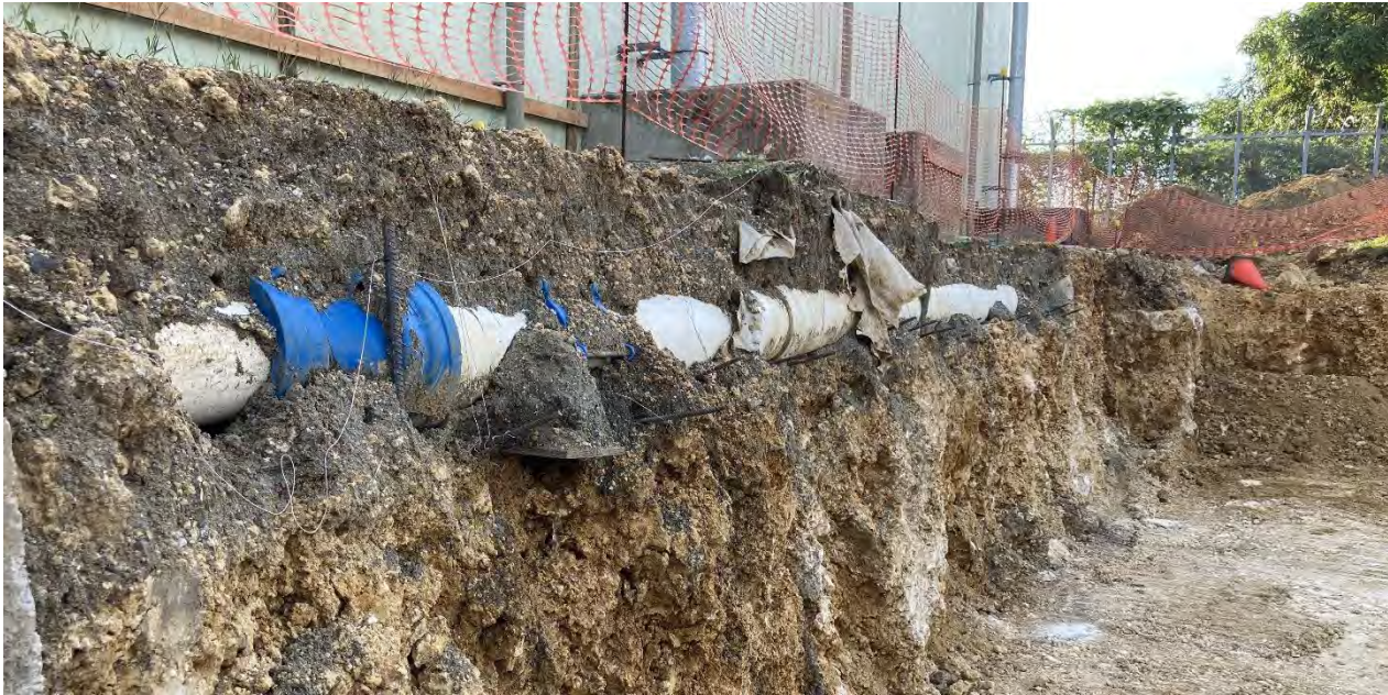
Figure 4 Exposed water main during excavation at Tasahe reservoir site (18/04/23)
