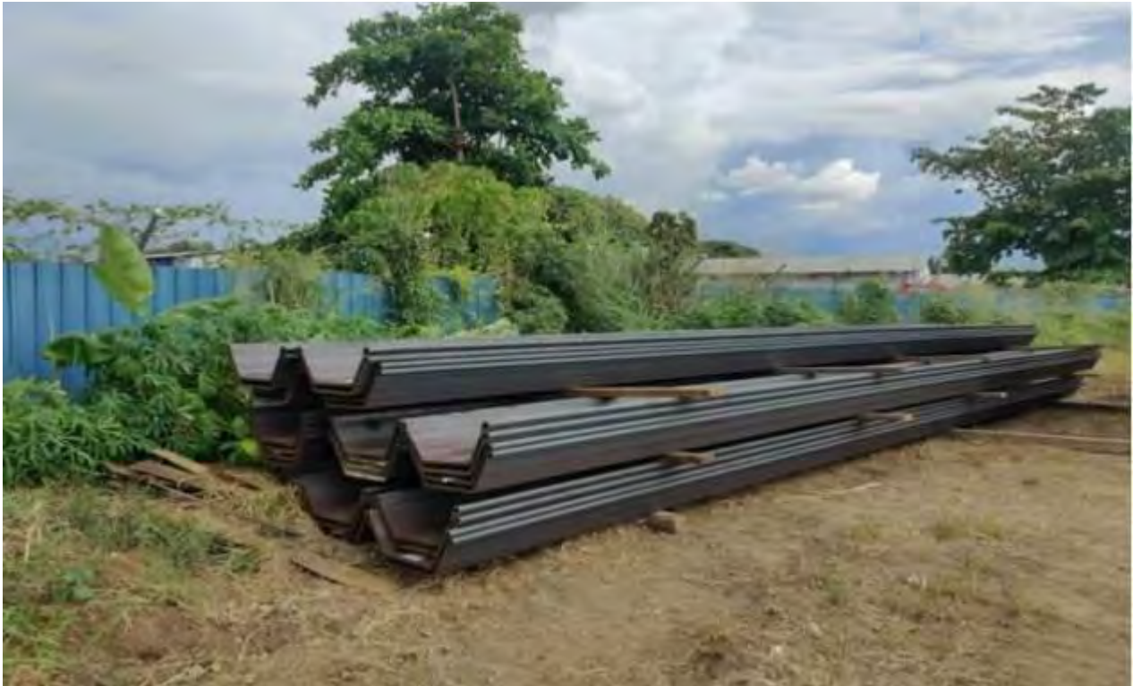
Figure 7 Ranadi Goodwood – Sheet piles on site (April 2023)
