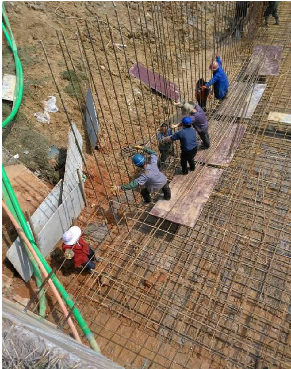
Figure 5: Local women building box-culvert for Fenggang River in 2017
