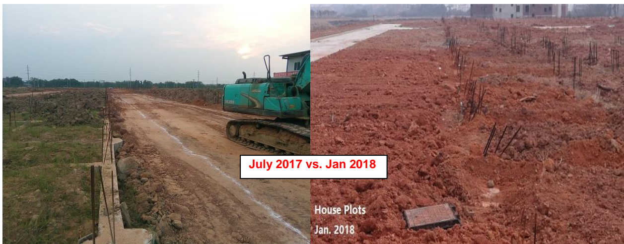
Figure 6: Construction Progress of Xianxi Relocation House Plots
