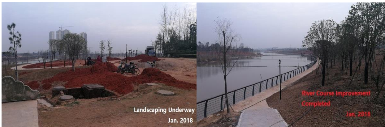
Figure 3: Construction Status of Fenggang River Component
