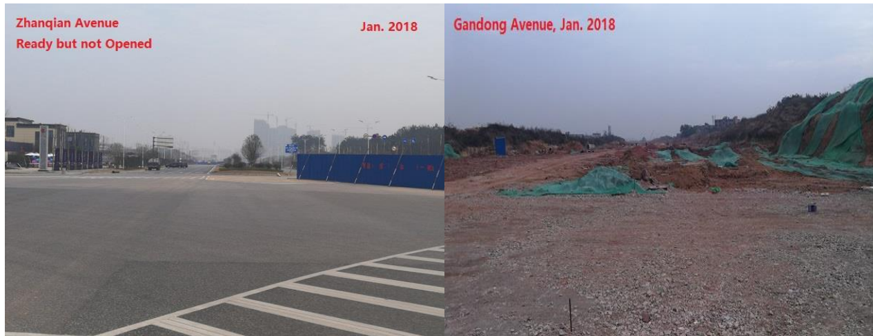
Figure 2: Construction Progress of Access Roads
