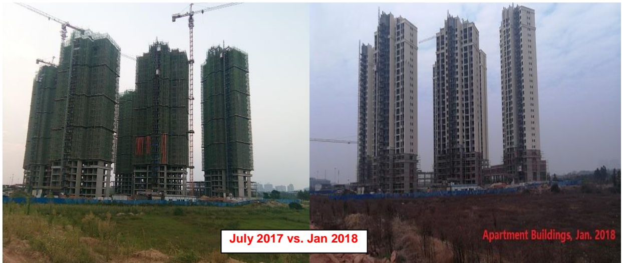
Figure 5: Construction Progress of Relocation Apartments
