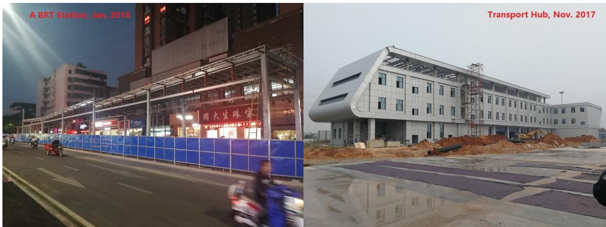
Figure 4: Construction Progress of Transport Hub and BRT
