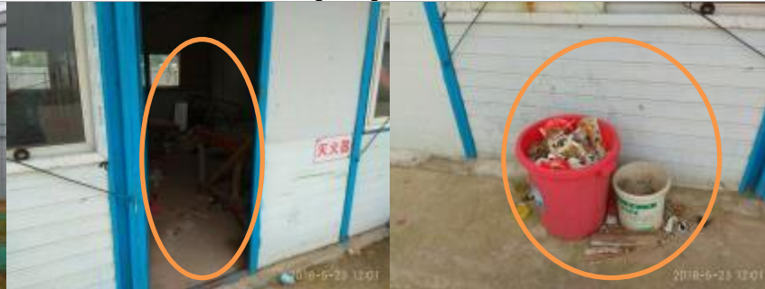
Contractor's camp garbage randomly disposed
