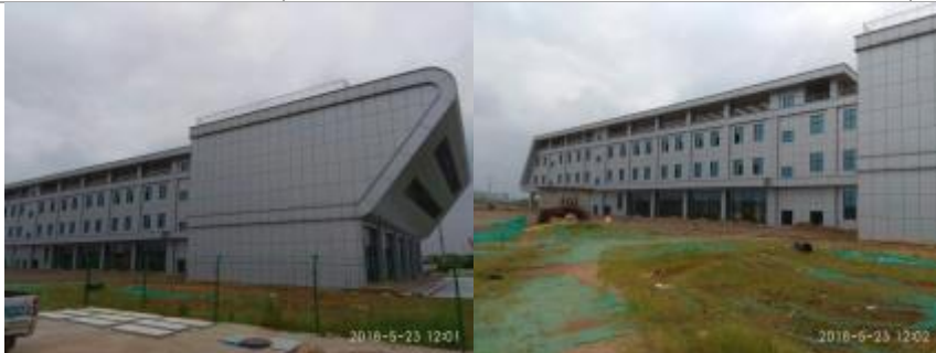
Main structure completed
