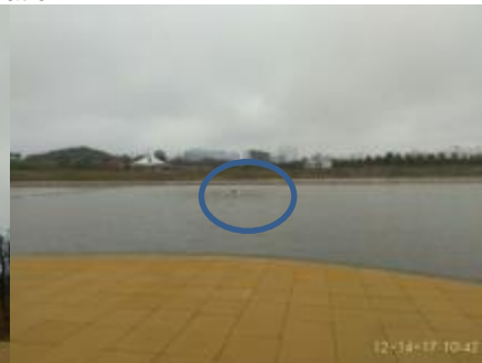
Water purification facility (aerobic)
