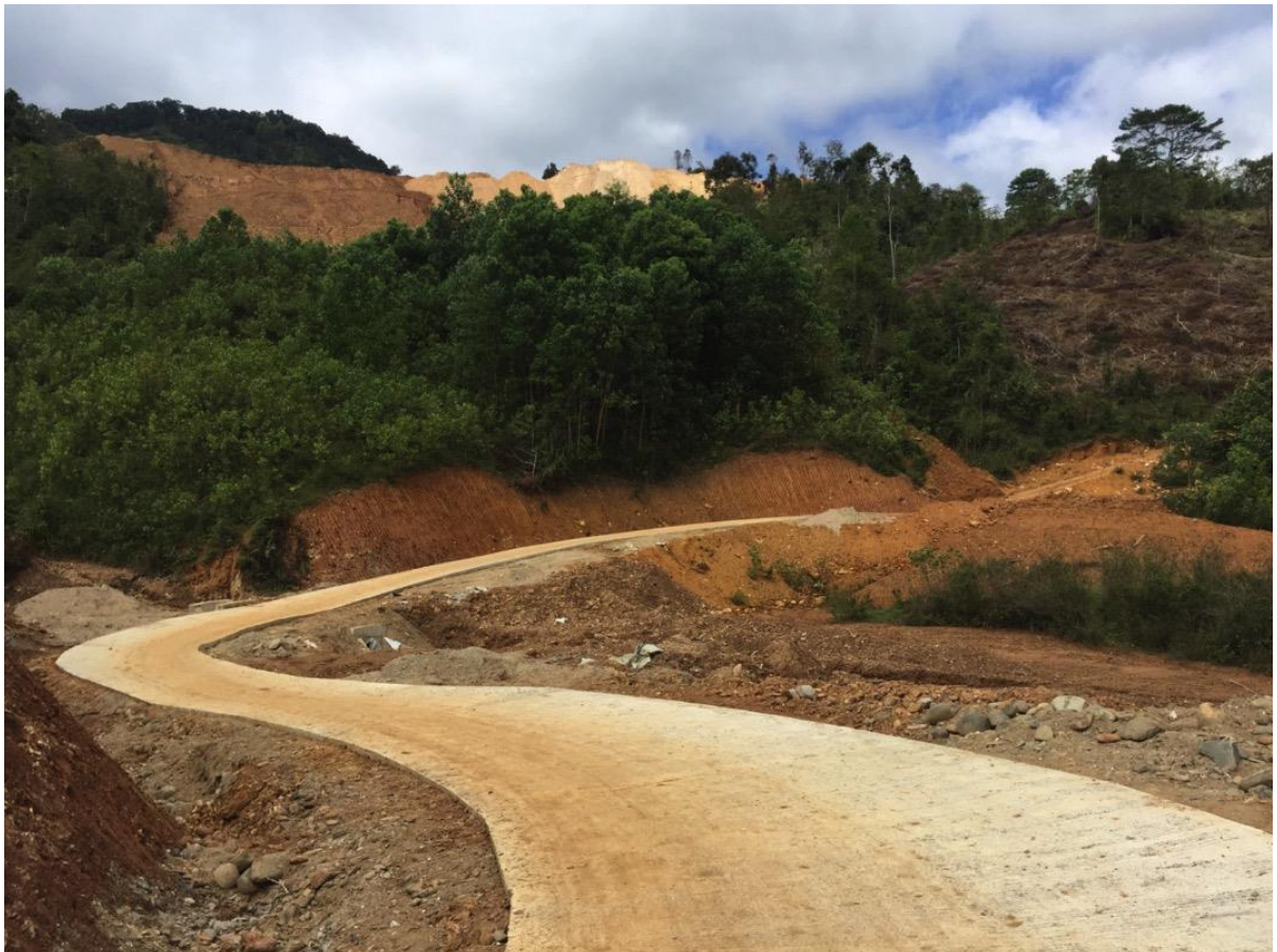
Figure 2 - Construction site at A Banh 2 road subproject
