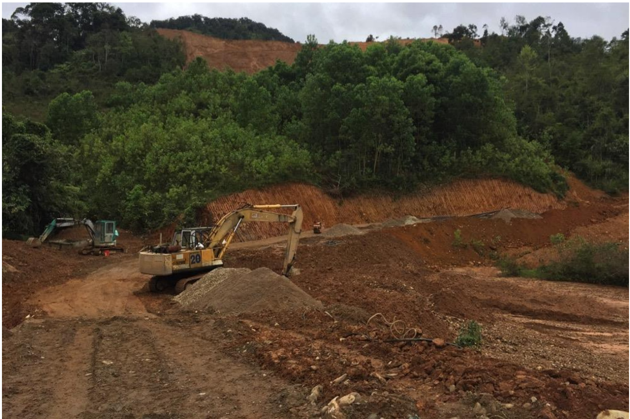
Figure 2 - Construction site at A Banh 2 road subproject
