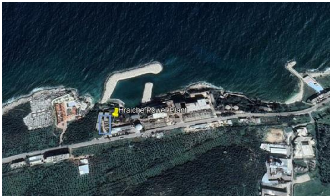
Figure C-2: Aerial view of Hraiche power plant with marked position of the transformers storage site
