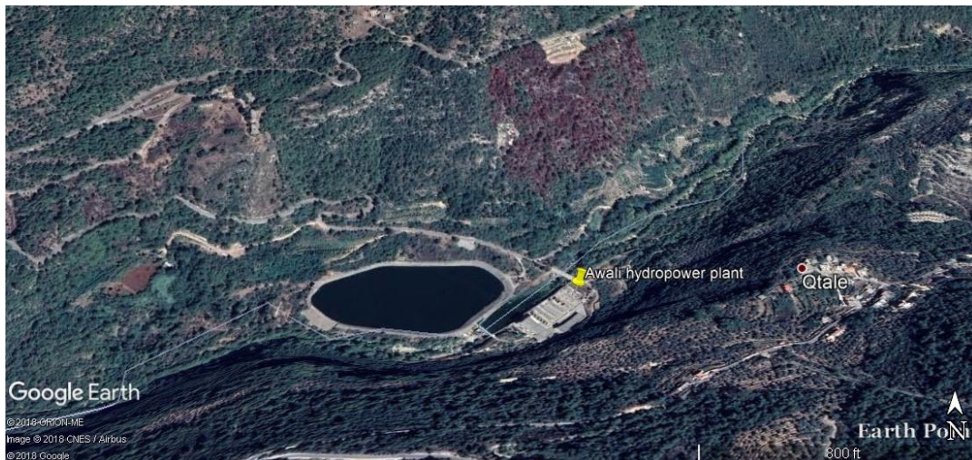
Figure C-12: Awali hydro power plant
