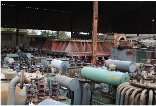
View of transformers stored at the site
