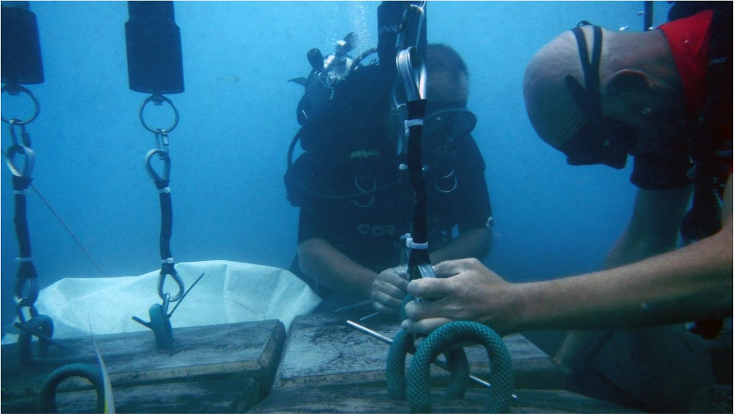
The SSB is composed of an array of multiple vertical tubes (SSB units) that mimic the visual effect of a natural kelp forest, which sharks tend to avoid so as not to get entangled. Kelp is a type of algae that attaches to the seabed and grows to the water's surface, forming a dense curtain.
