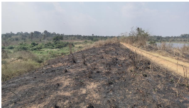
Figure 5-1.2 Dam Height of Aisegba Reservoir
