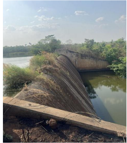
Figure 5-2.3 Spillway of Itapaji Reservoir
