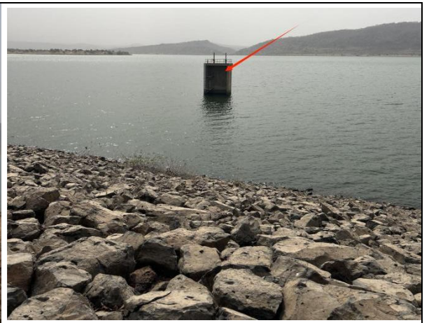
Figure 3-3 Water Transmission Gate of Balanga Reservoir
