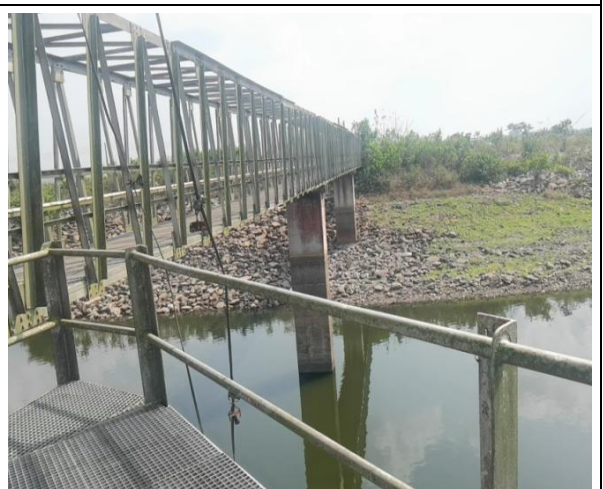
Figure 4-6 Access Bridge of Water Transmission Gate of Owena Reservoir
