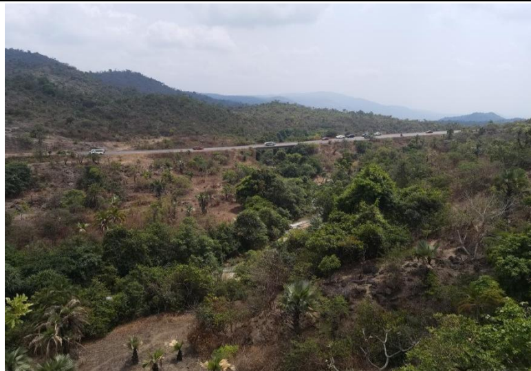
Figure 6-1.5 Proposed Dam Site of Asop Falls Hydropower Project
