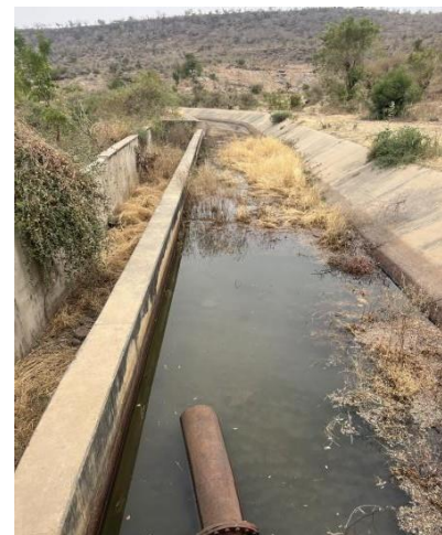
Figure 3-5 Water Transmission Channel of Balanga Reservoir
