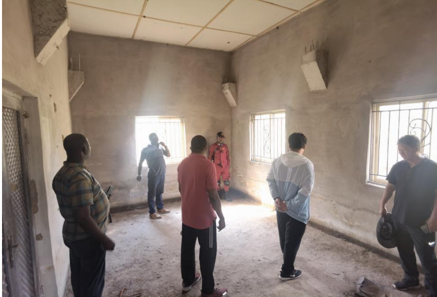
Figure 5-2.1 Powerhouse of Itapaji Hydropower Project Built
