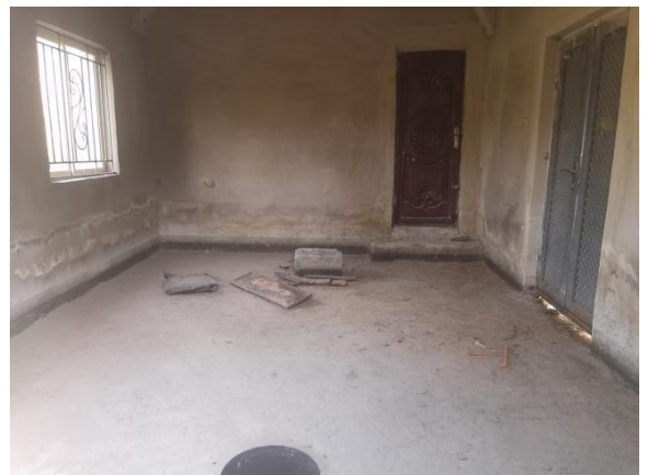
Figure 5-2.7 Inside the Powerhouse of the Proposed Hydropower Project of Itapaji Reservoir
