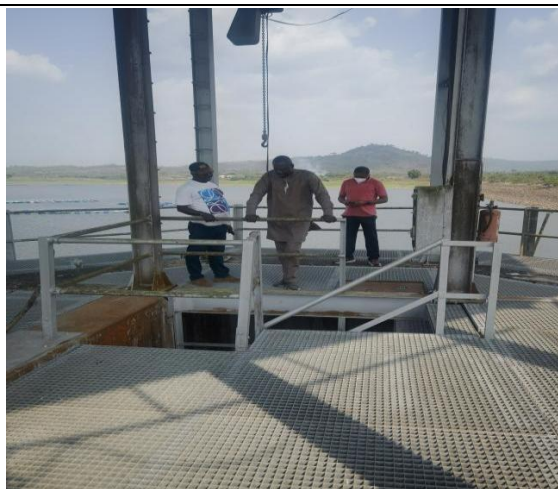
Figure 4-5 Water Transmission Gate of Owena Reservoir
