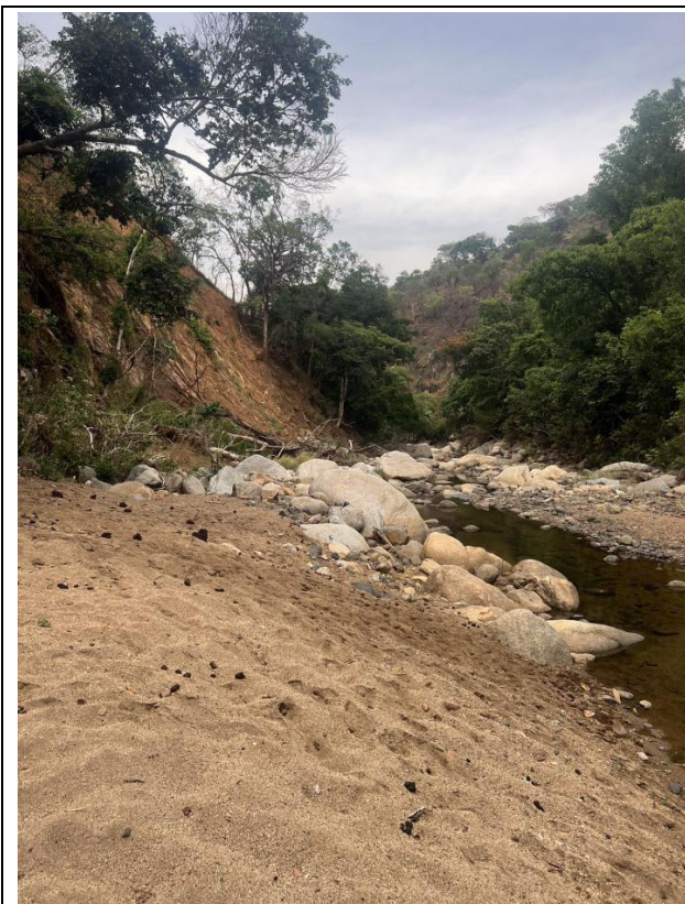
Figure 7-3.7 Upstream River Channel of Mayo Selbe 3# Hydropower Project
