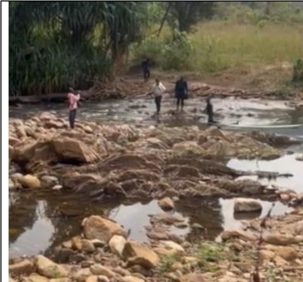
Figure 7-2.7 Site Visit to Mayo Selbe 2# Hydropower Project
