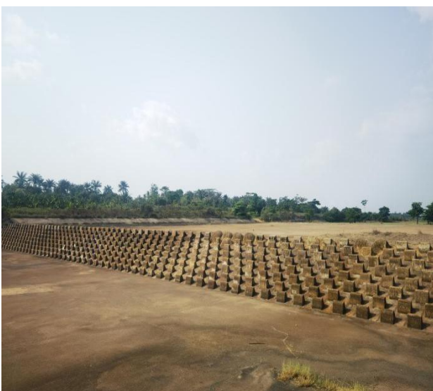
Figure 4-11 Spillway of Owena Reservoir
