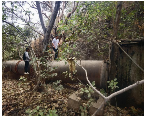
Figure 3-9 Site Visit to Pipeline of Balanga Reservoir
