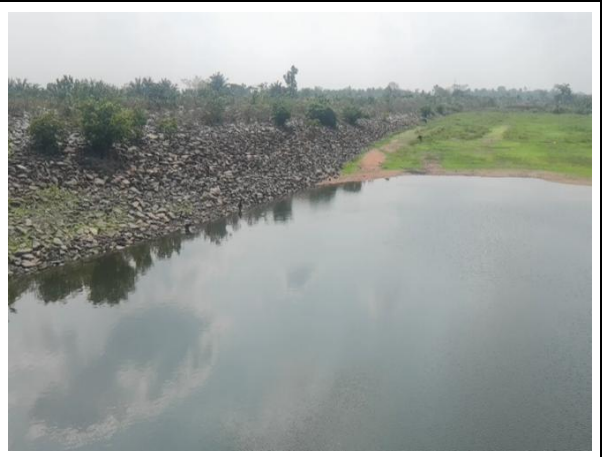
Figure 4-4 Upstream Dam Slope of Owena Reservoir
