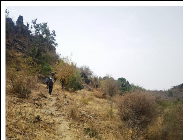
Figure 3-8 Site Visit to the Dam of Balanga Reservoir
