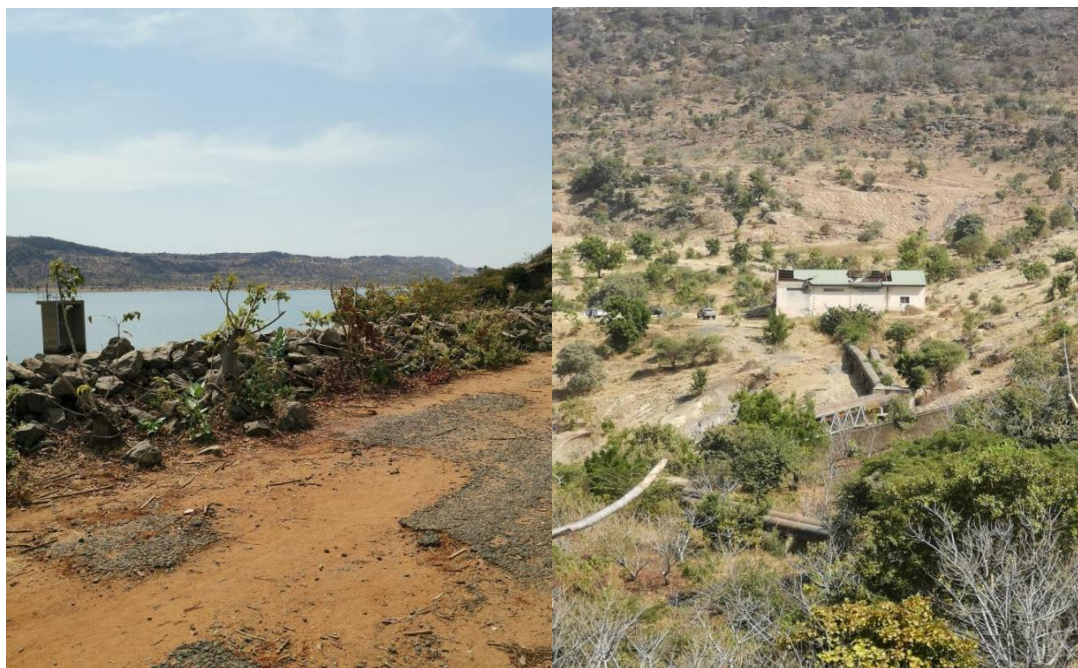
Fig 1.3. Photo of the site at the dam crest and along the water conveyance pipe
