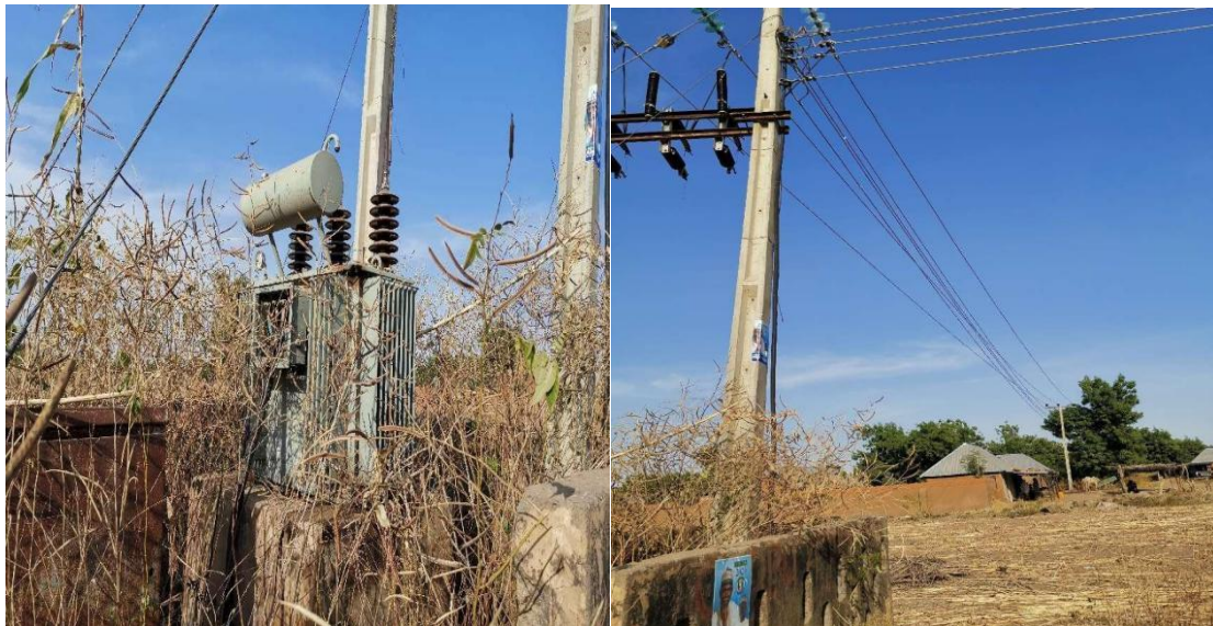
Fig 1.11. Investigation of Existing grid
