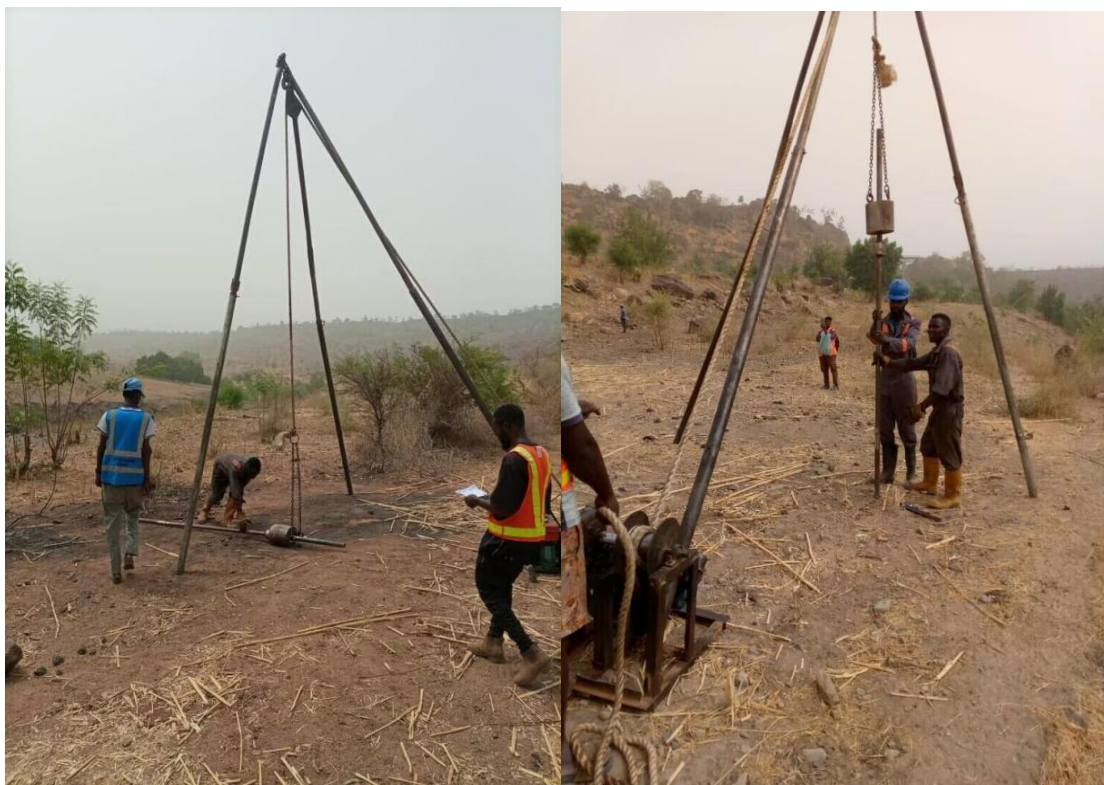
Fig 1.5. Geotechnical exploration work
