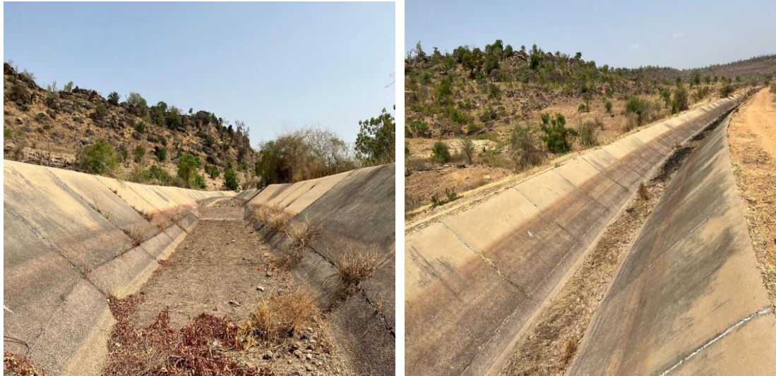
Fig 1.8. Investigation of existing irrigation channel
