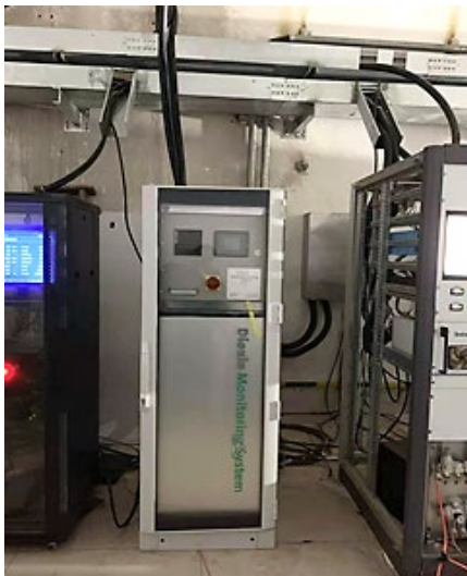
Figure 6. Continued Dioxin Emissions Sampling at Everbright Incinerator (Ningbo)
