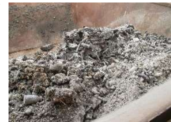
Figure 79 Evidence of not fully incinerated residue of medical waste
