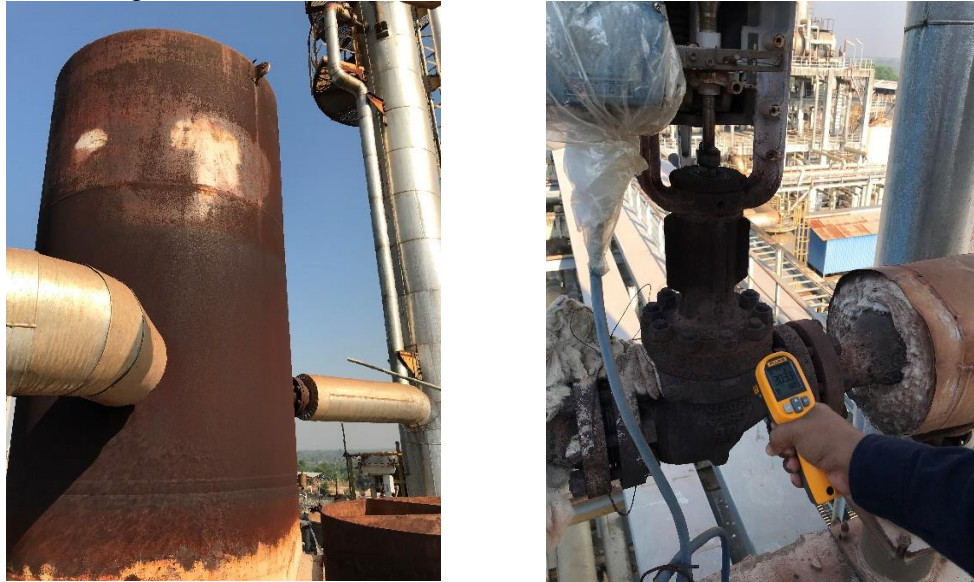
Figure 8: The Steam Vent stacks and the Vent Control Valve
