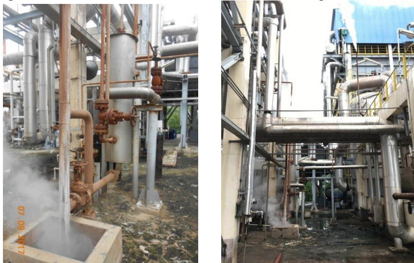
Figure 11: The B/D hot-well and flash steam venting from blowdown water
