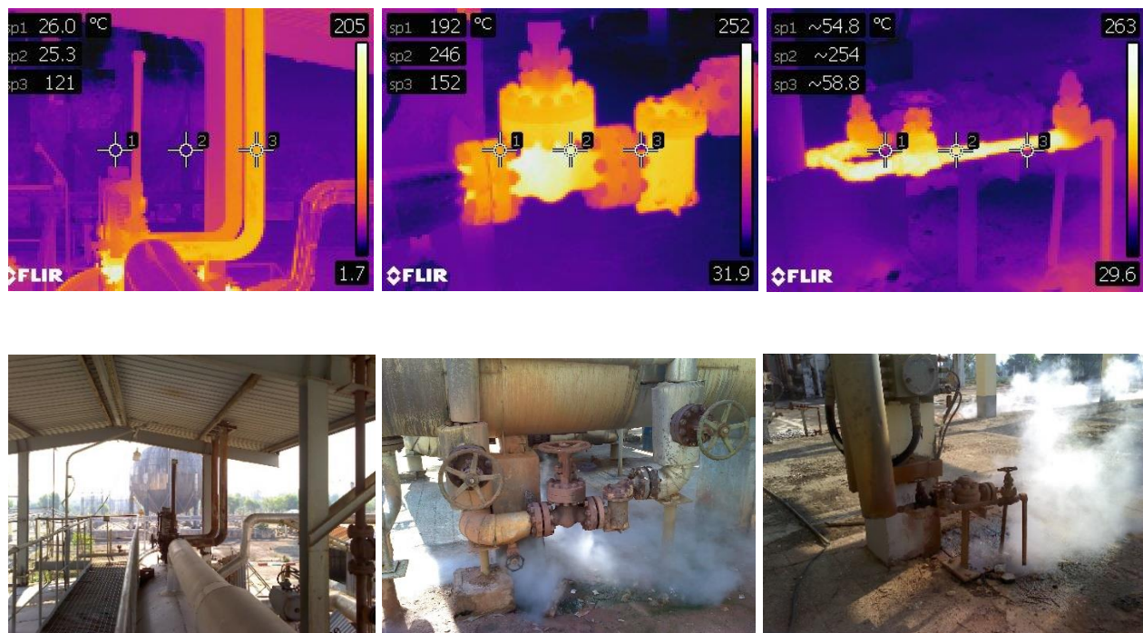
Figure 6: Leaking Relief Valves at B-4001, Flange & Steam Trap at the 5.0 MPa header
