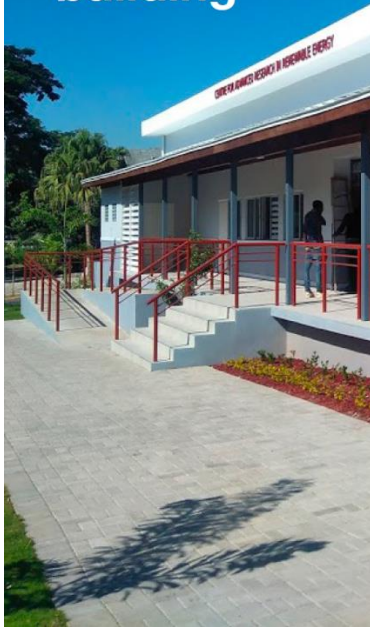
Building façade (showing shading, treatment of openings, window-to-wall ratio, foliage, light coloured exterior)
