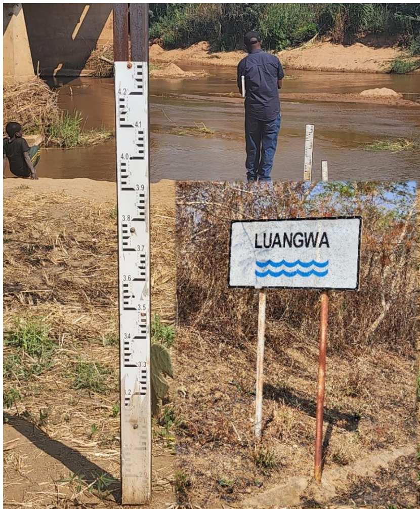
Photograph 3: Gauge plates at Kampumbu Bridge on the Luangwa River
