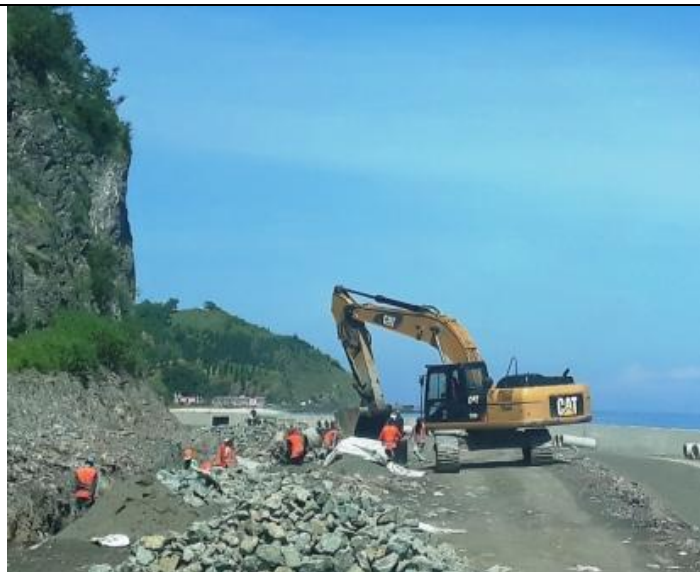
April 2019, workers are equipped with PPE constructing the line drain at Sta 10+200 L/S
