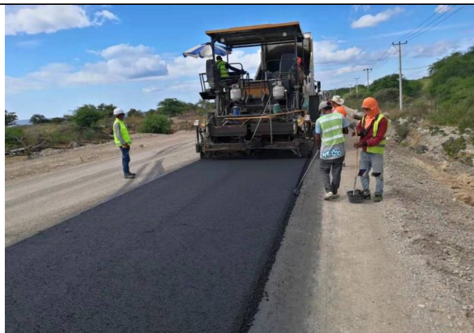
June 2019. Asphalt Paving Sta. 115+360 R/S workers are provided with PPE.
