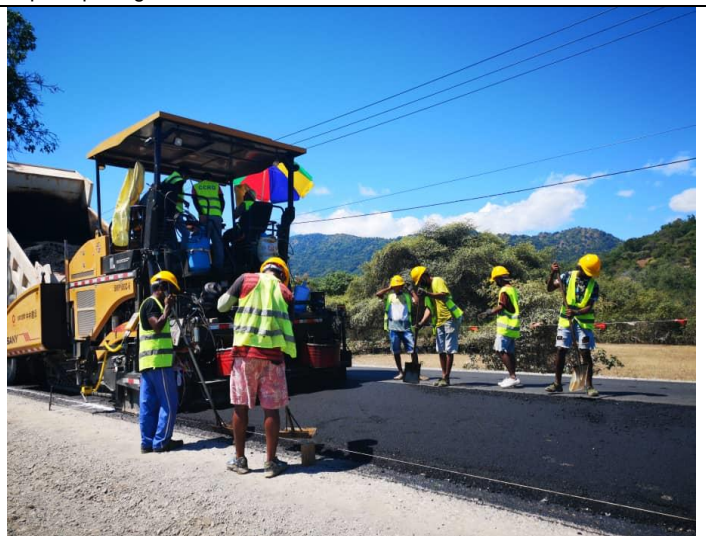
May 2019 (Sta. 108+800) worker are not provided with PPE during the asphalt paving work.
