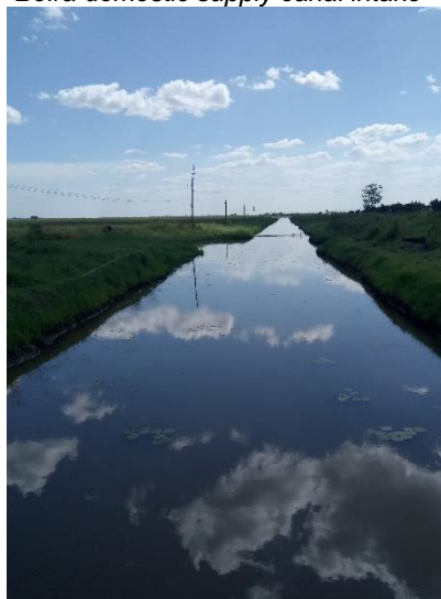
Beira domestic supply canal intake
