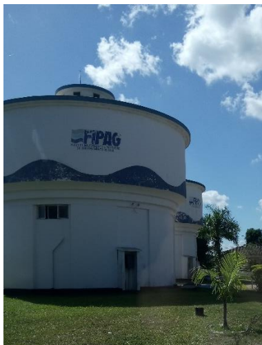
Beira domestic water treatment plant
