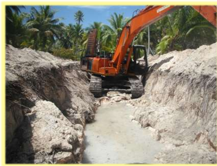
Excavation of groundwater abstraction gallery.
