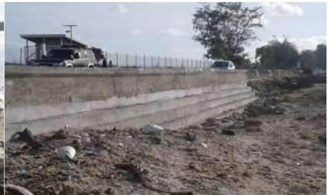
Coastal protection works at Site 2 (Nanikai—Tearaereke causeway). Left: before showing breaches in existing wall; Right: nearly completed gravity concrete wall before reinstating the beach.
