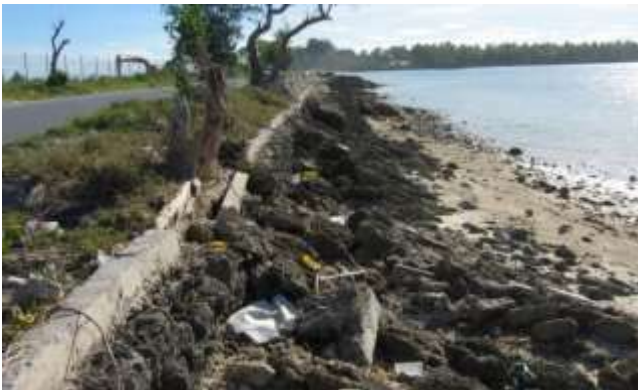
Coastal protection works at Site 2 (Nanikai—Tearaereke causeway). Left: before showing breaches in existing wall; Right: nearly completed gravity concrete wall before reinstating the beach.
