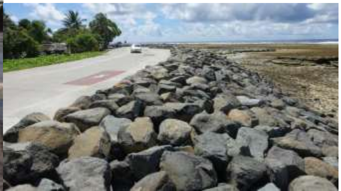
Coastal protection works at Site 10 in Temaiku designed and construction funded under KAP III (by the KRRP civil works contractor). Left: before showing erosion and diversion of road; Right: completed works designed for a 50 year return period event with sea level rise.
