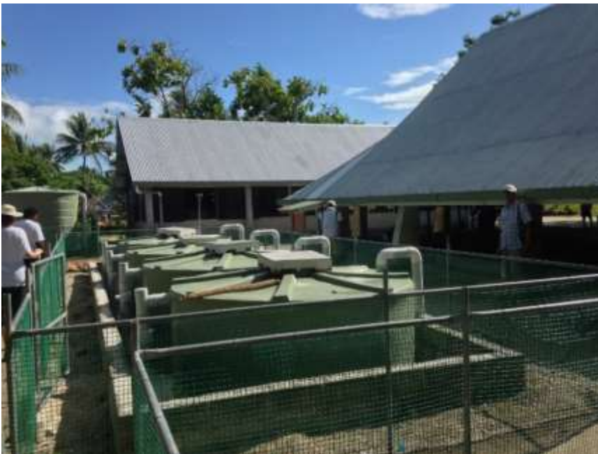
Water storage tanks as part of the Tabonibara rainwater harvesting system in North Tarawa. Water is collected from the roof of the adjacent maneabwa.
