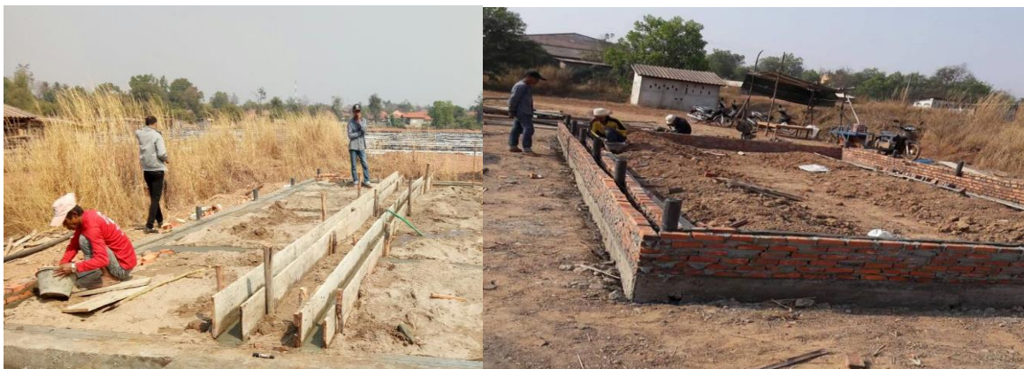
Preparation of foundation at Khok Saath salt factory
