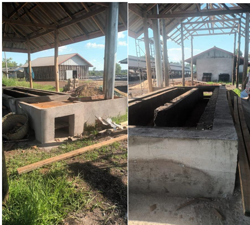
Figure 24: Construction of pellet furnace at Veunkham salt factory
