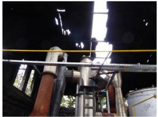
The air pollution control system under a leaking roof
