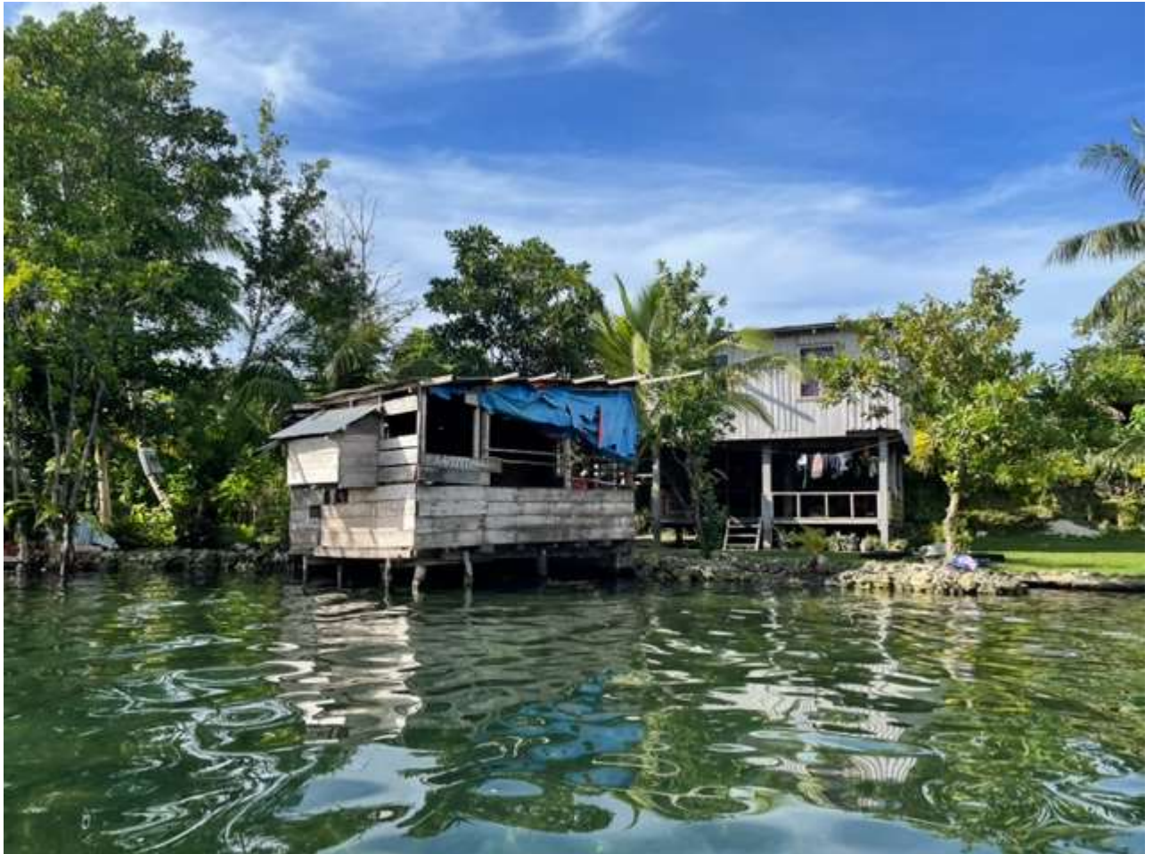
FIGURE 17: HOUSE OVER STILTS BUILT FROM MANGROVE WOOD
